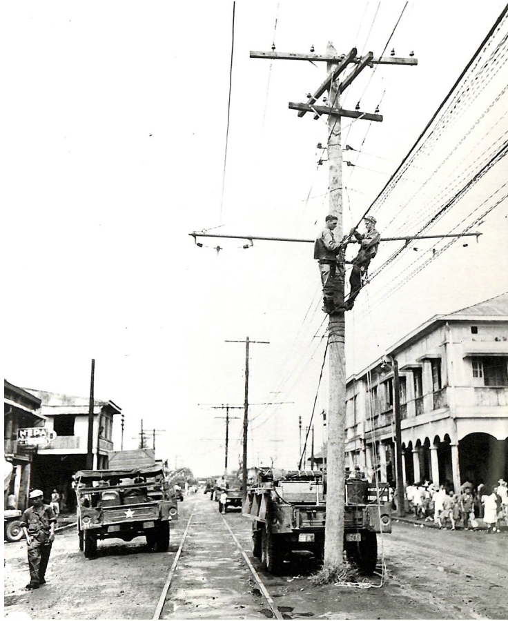
Figure 20. US Army Signal Corps Wire Crew Strings Heavy Communication Wire (February 11, 1945).
