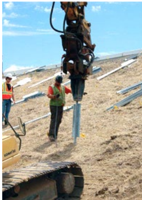
Figure 3. Platepile installation (McCormick 2014).
