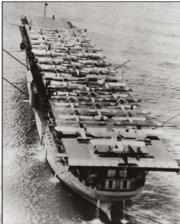
USS Langley, the Navy's First Aircraft Carrier - Converted in 1920 from the collier USS Jupiter (AC-3), she was attacked by Japanese bombers in February 1942, was badly damaged, and had to be scuttled by her escorts.
