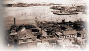
AERIAL VIEW OF DOWNTOWN NEWPORT AND NTS
