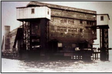
Gould Island Firing Pier
