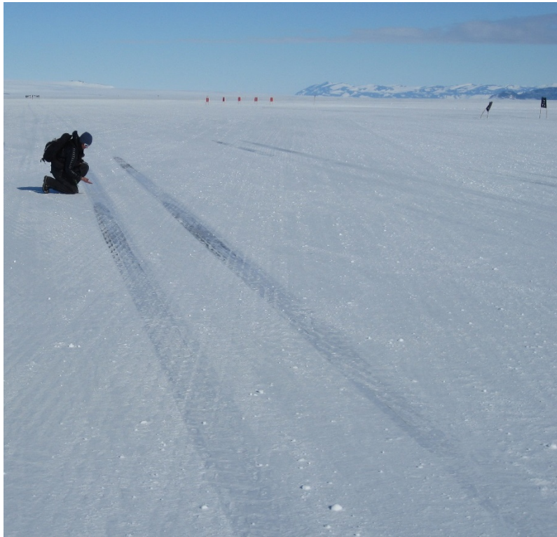
Figure 66. Tracks of eroded rubber from a C-17 landing.
