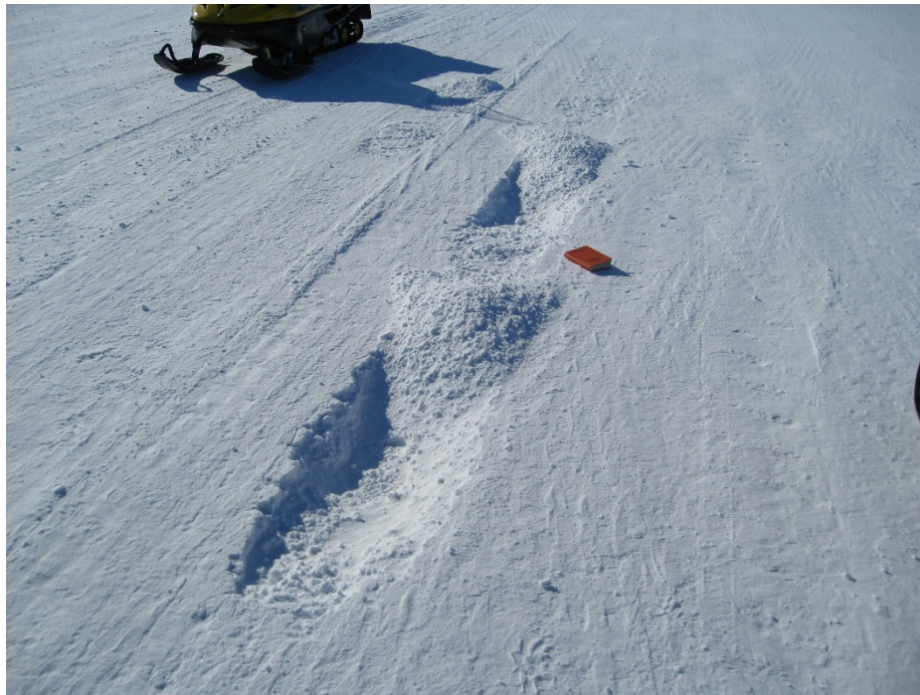
Figure 70. Isolated but deep ruts associated with one tire path of the main landing gear at the point of C-17 rotation at takeoff.
