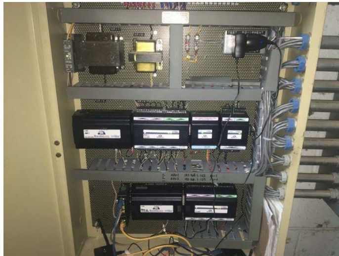
Figure 16. Retrofit AHU Controls
