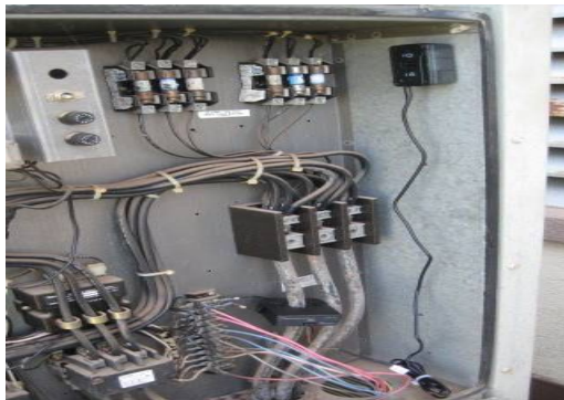
Figure 14. Chiller Power Measurement
