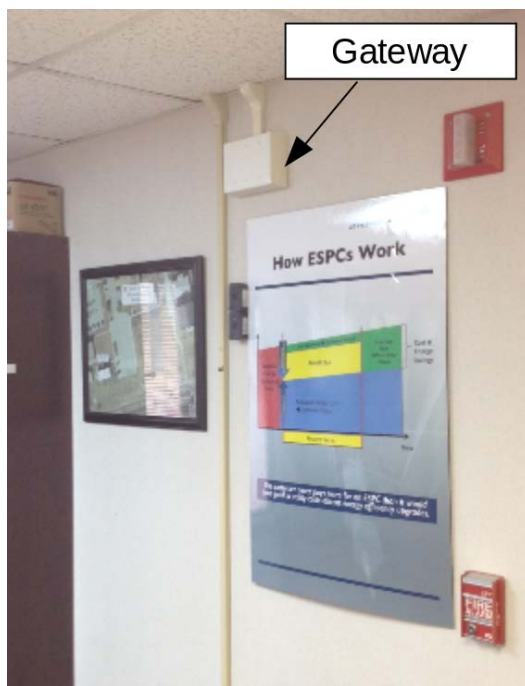
Figure 28. Typical Gateway Mounting
