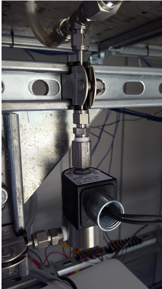
Figure 15. Omega SV133 normally open fluid control valve.
