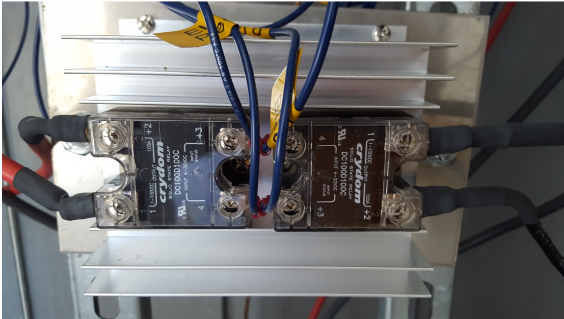
Figure 12. Crydom solid state relays used for electrolyzer control.
