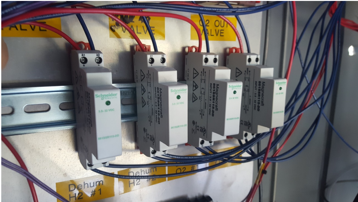
Figure 13. Magnecraft relays for control of dehumidifier power.
