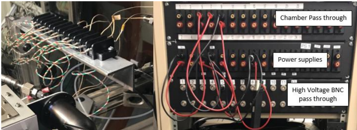
Figure 9: Chamber patch panels interior (left), exterior (right)
