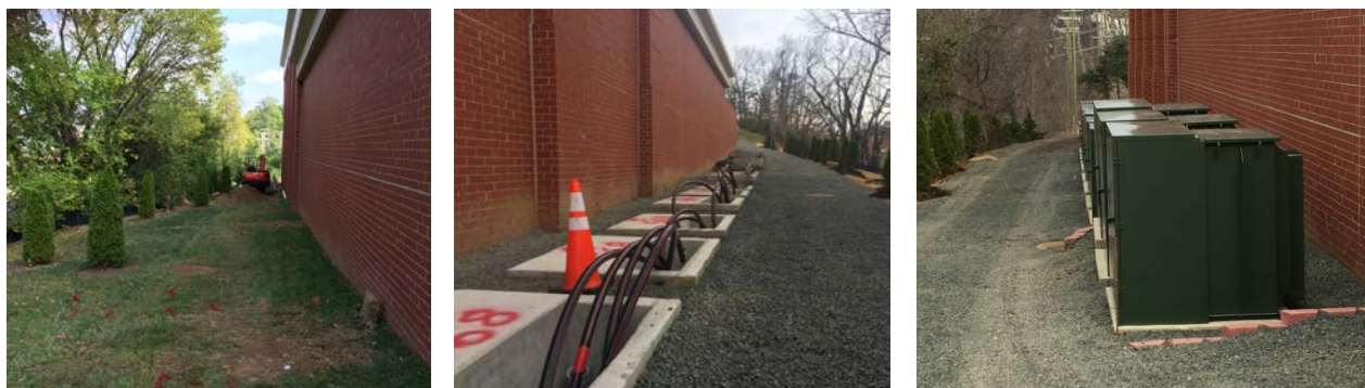
Figure 30. Single Phase Voltage Regulation Equipment Site Installations Conditions Prior, During, and at Completion on March 2016
