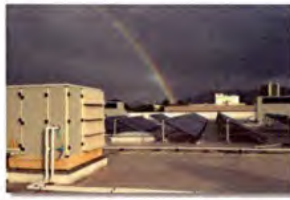
(b) (above) a AILR LD unit was installed at a supermarket in Hawaii. The process heat for desiccant regeneration was supplied by solar thermal system.
