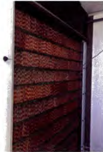
The AILR patented absorber and regenerators design. Cooling tube are imbedded into an evaporative medium
