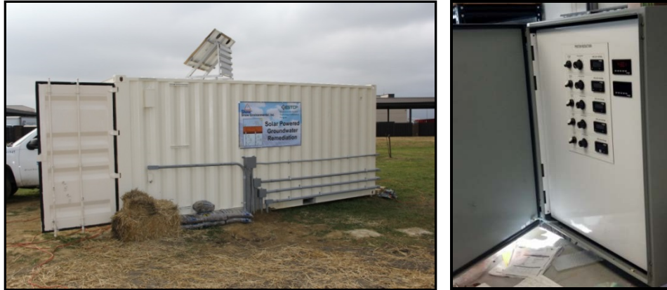
Figure 5.6. Conex Box and PRT Control Panel
