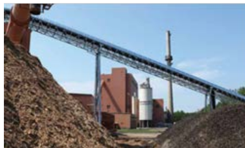
Figure 12. RE Energy Facility on Ft. Drum
