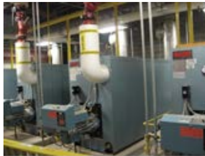
Figure 11. The Smith Boilers
