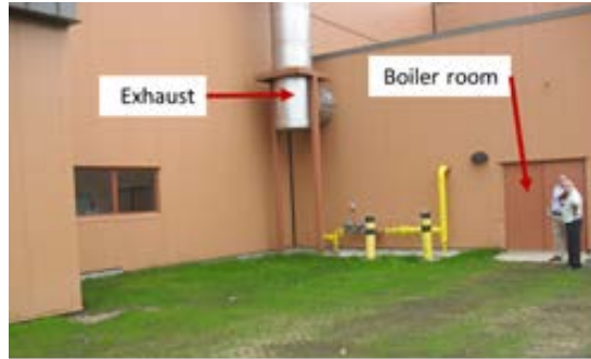
Figure 10. Close of Installation Area
