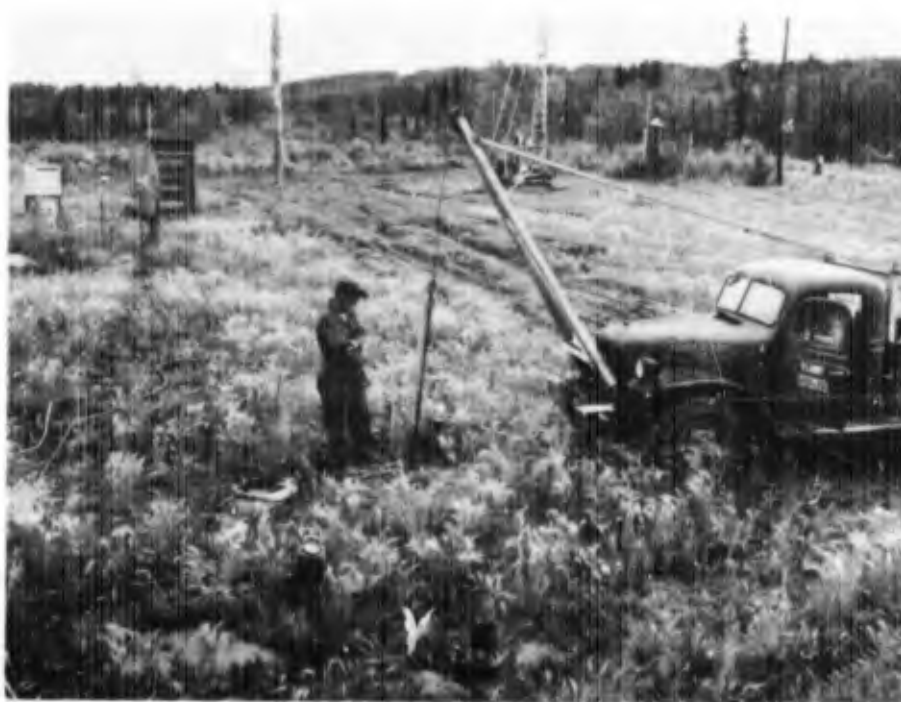
Figure 57. Removing Shelby tube with truck winch and A-frame.
