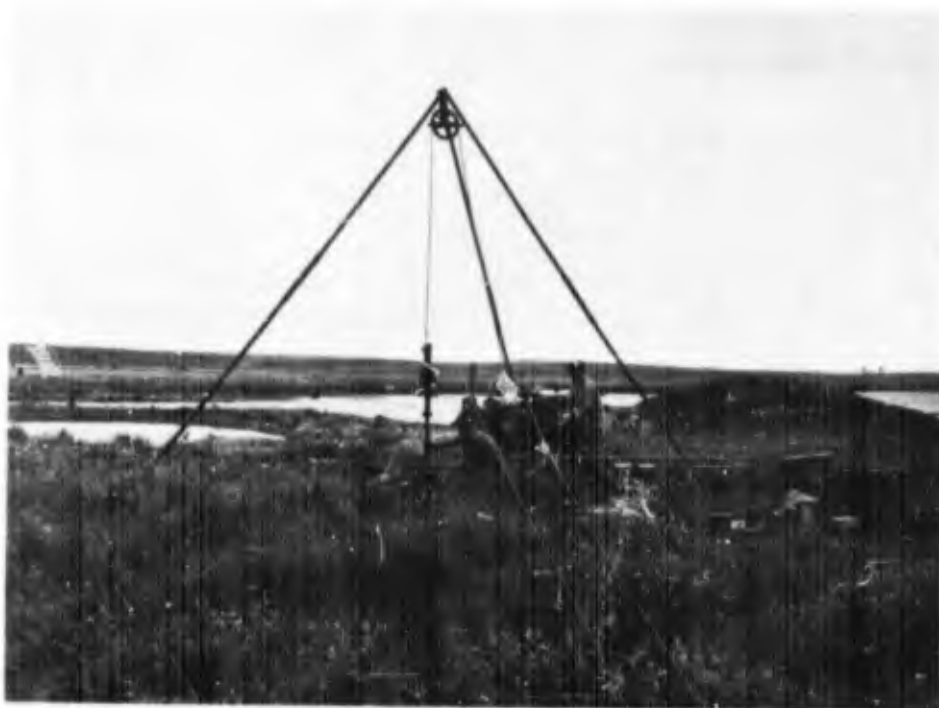
Figure 31. Drive sampling with Chicago Pneumatic core drill.
