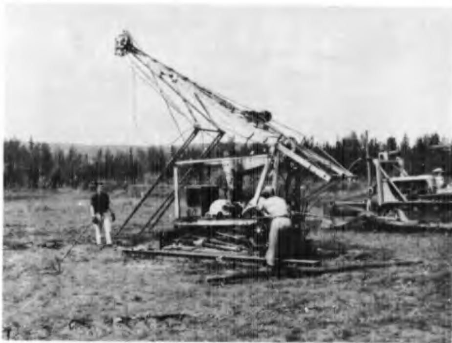
Figure 11. Lowering tower of Cyclone drill for movement.
