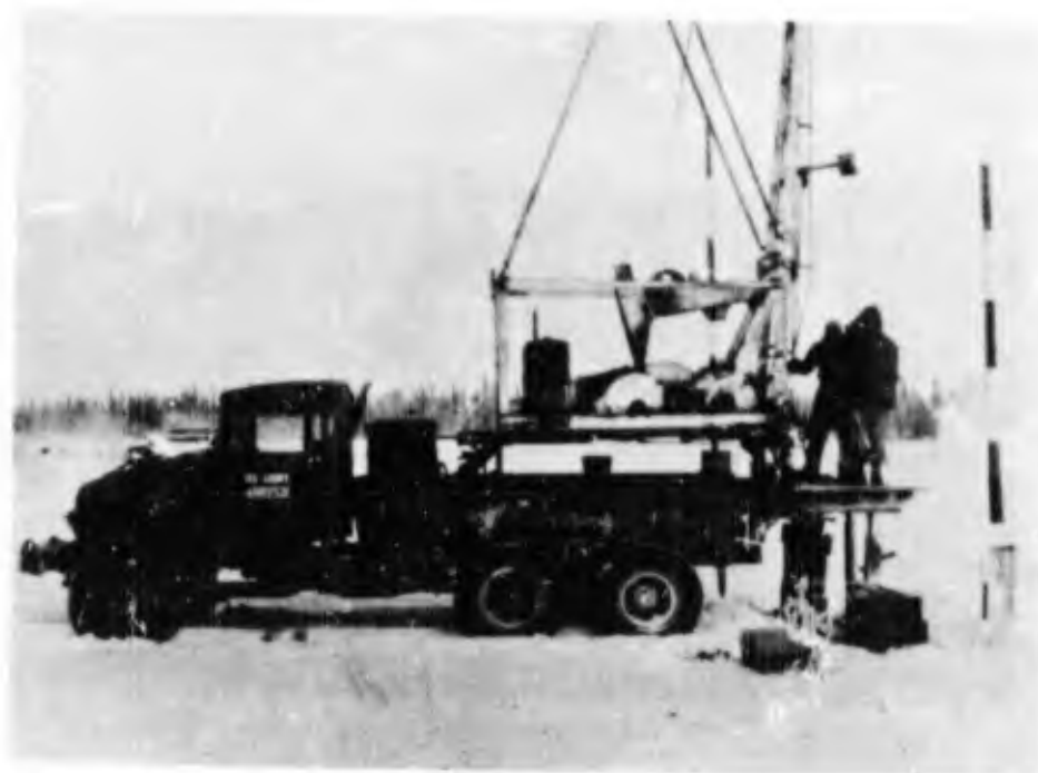
Figure 10. Cyclone drill in use while mounted on 2½-ton truck.
