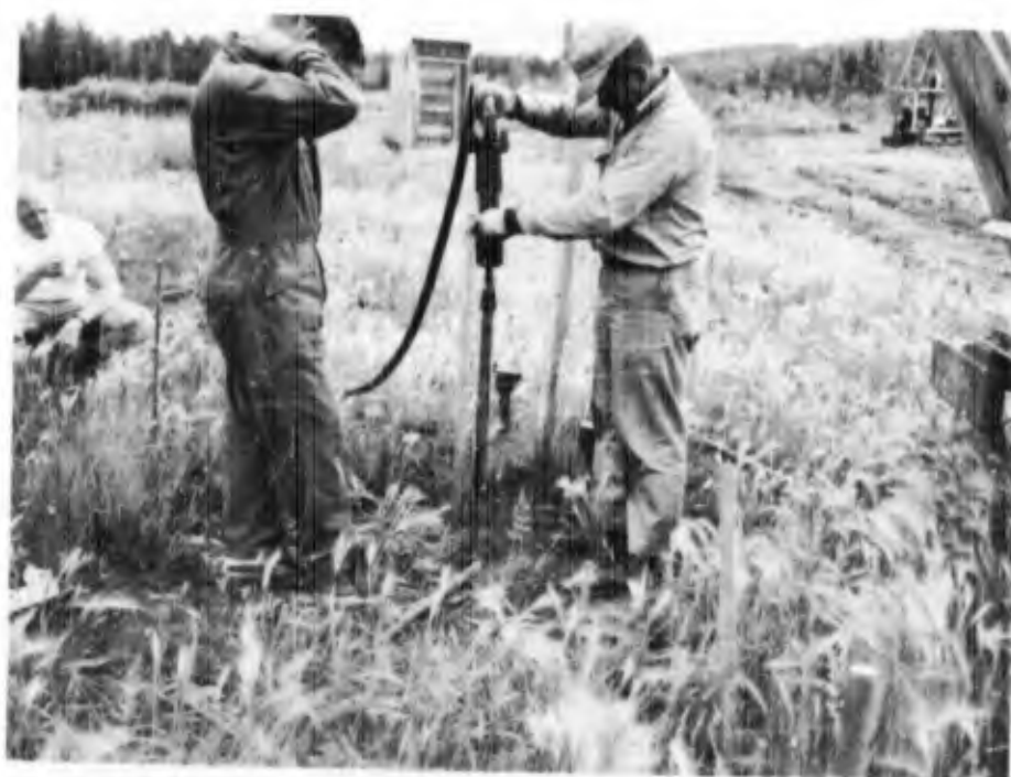
Figure 56. Driving Shelby tube with pavement breaker.
