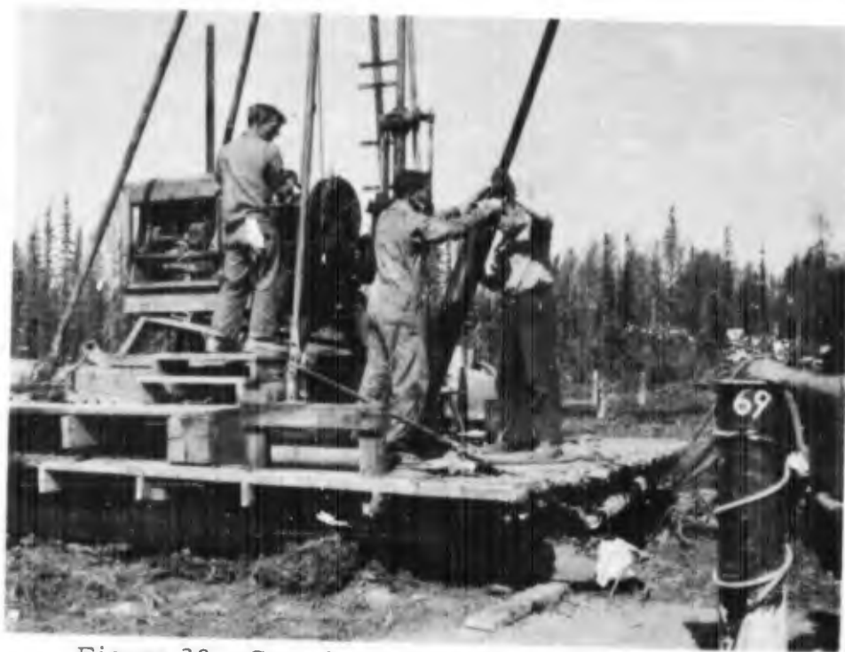
Figure 20. Core barrel used with Longyear drill.
