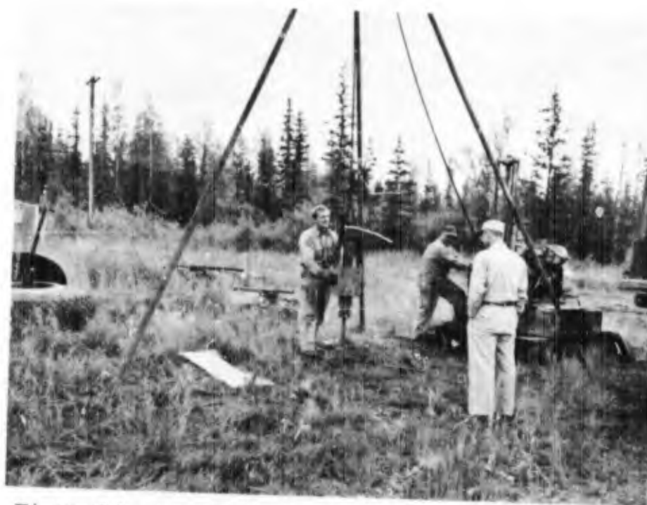
Figure 50. Driving Shelby tubes with Acker core drill.
