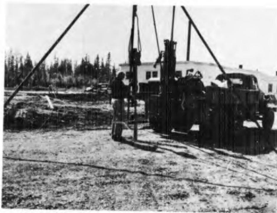
Figure 29. Drive sampling with Acker core drill.
