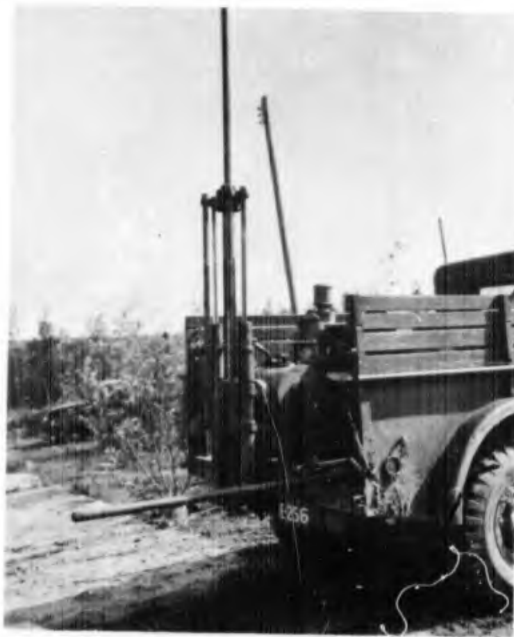
Figure 26. Acker core drill mounted on 3/4-ton truck.
