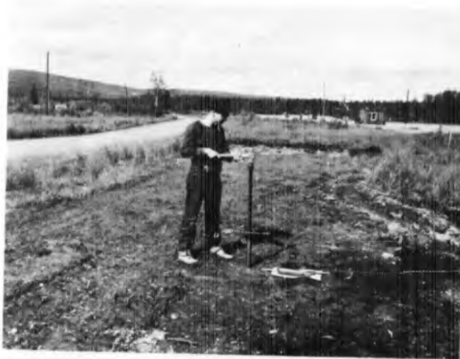
Figure 55. Driving Shelby tube with sledge hammer.
