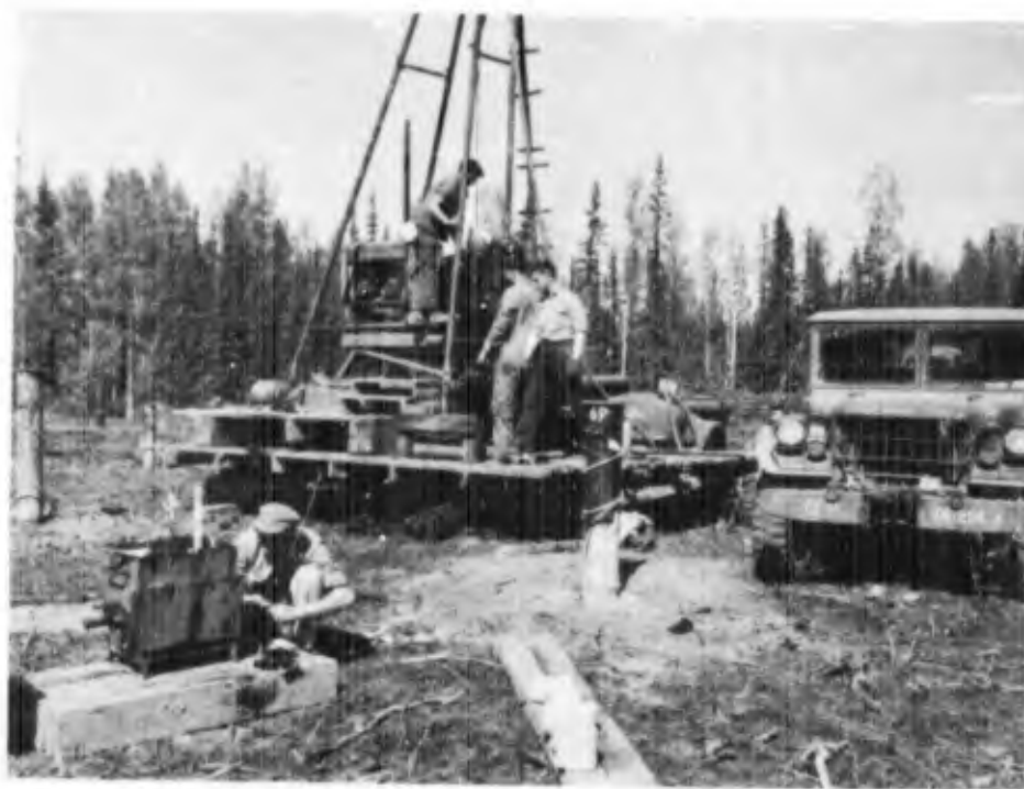
Figure 18. Longyear core drill on timber platform.
