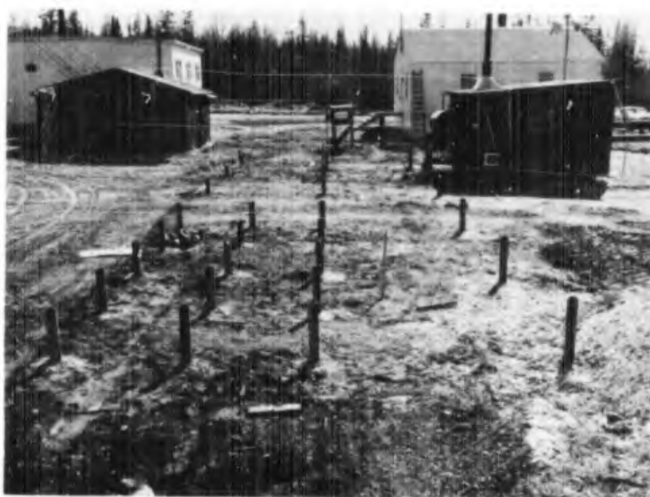
Figure 16. Steel pipes used as foundation piles.
