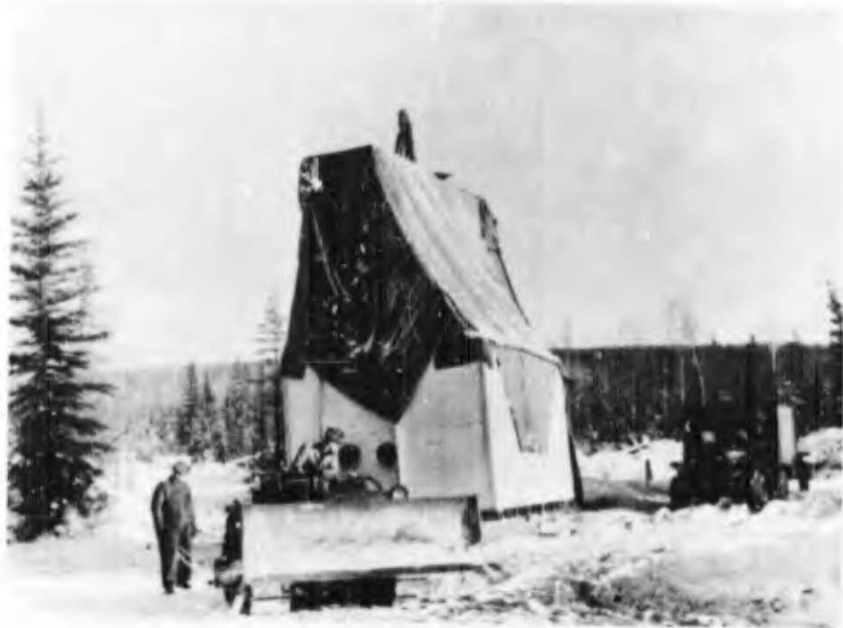
Figure 19. Longyear drill with timber housing.
