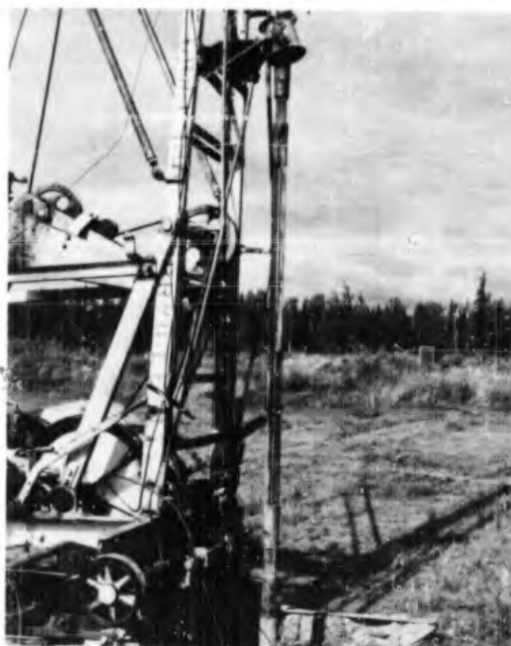
Figure 17. Drive sampling by use of jars.
