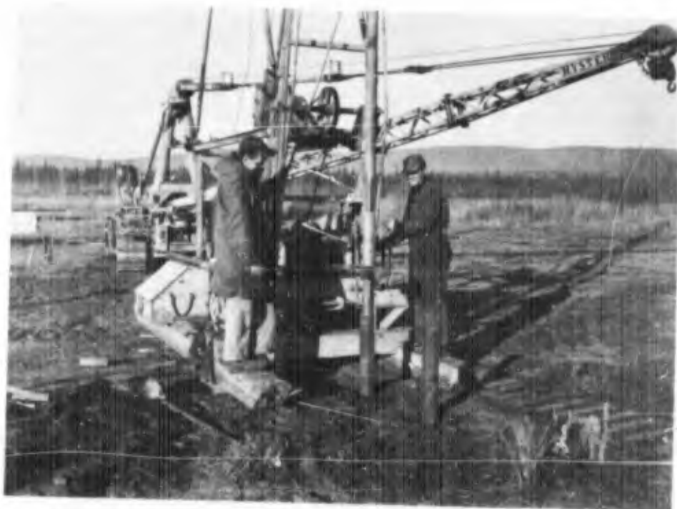
Figure 14. Pile driving with Cyclone churn drill.
