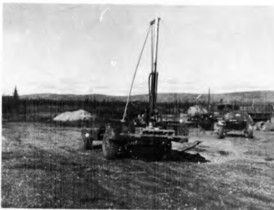
Figure 32. Concore core drill mounted on 3/4-ton truck.
