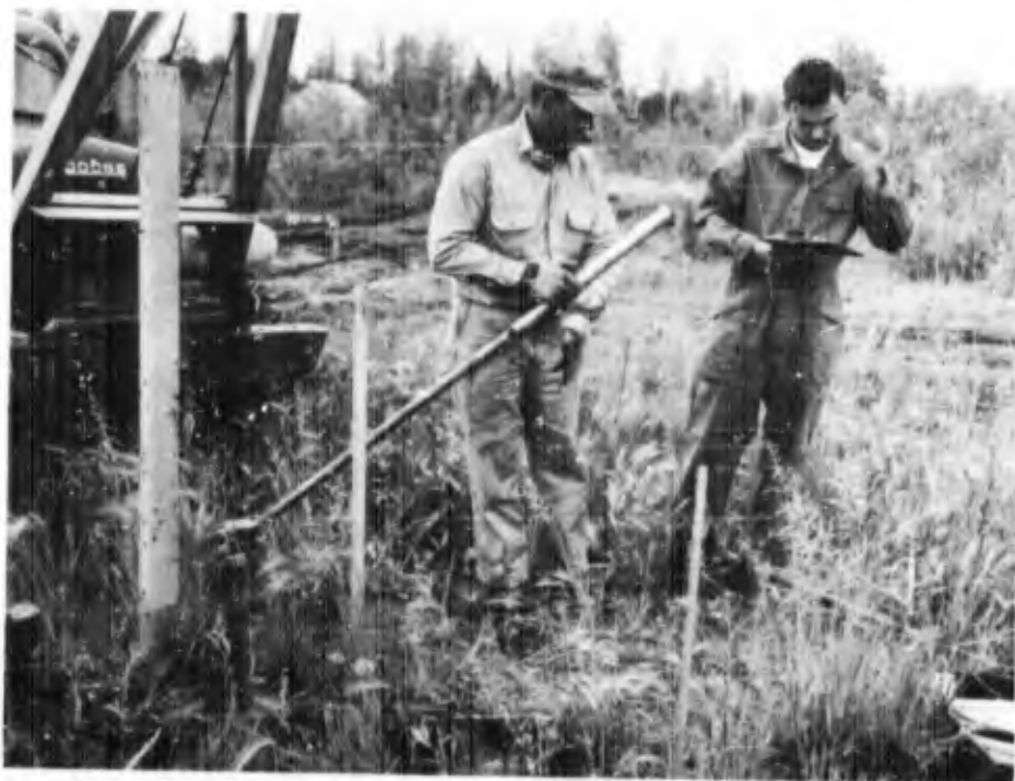
Figure 47. Thin walled electrical conduit sampler.
