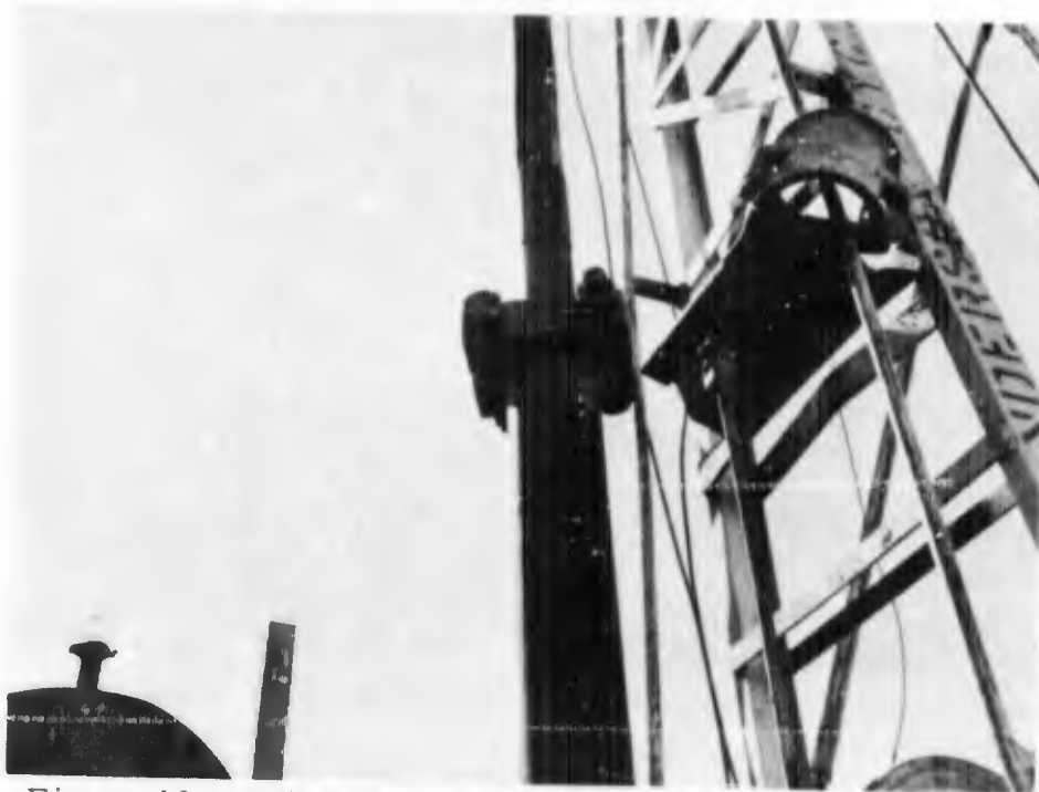
Figure 13. Drive clamps in position for driving casing.
