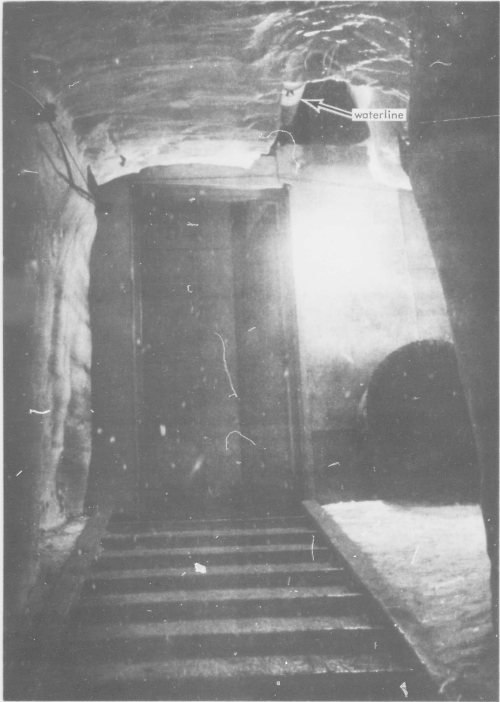
Figure 7. Typical passageway door showing bulkhead perforated by waterline and out-of-service ventilation fan.
