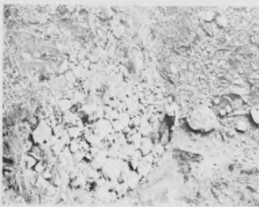
Photograph 8. Trinchera 18. Check Dam. Max. Height 12.3 Feet.
