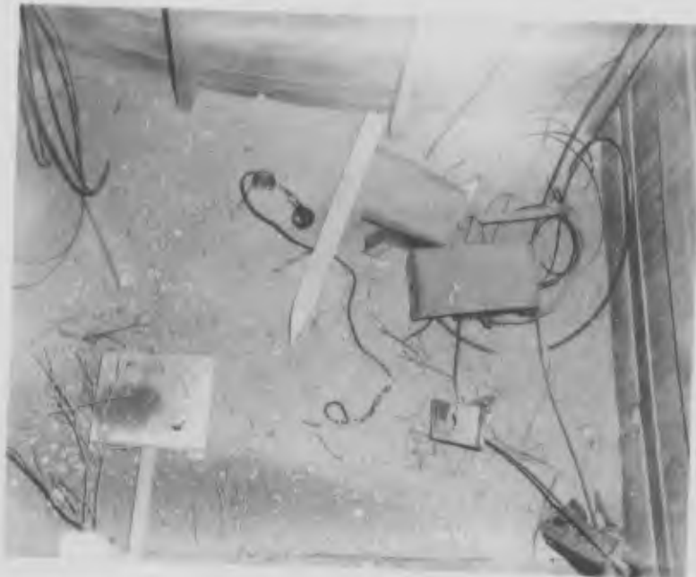
81 mm Mortar Position Before After
