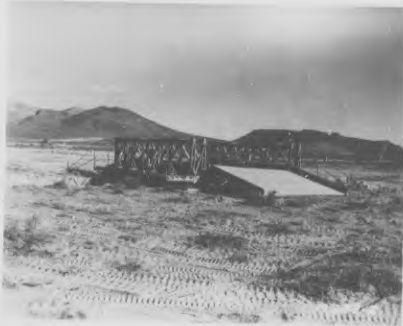
Bailey Bridge Before ↗ After ↘ Moved Sideways 5 Yards
