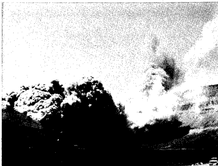
There was essentially no cloud rise. The sandbag stemming and the material scoured from the tunnel itself stayed close to the ground.
