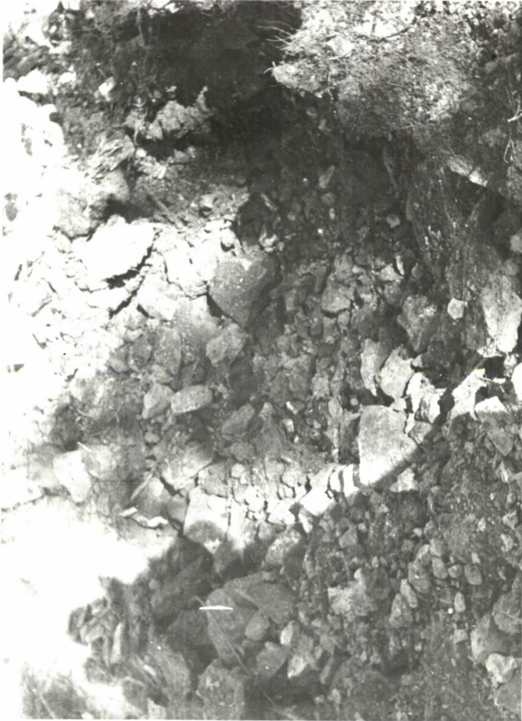
Fig 21 Shot #7: Result of 3 lb of liquid explosive in a 2 \frac{1}{4} " dia by 3' deep-bored shot hole
