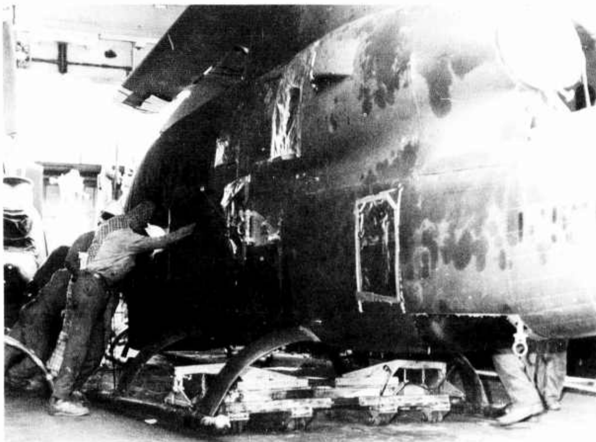
Figure 8-8. Helicopter Positioning Device (MTMC Device).
