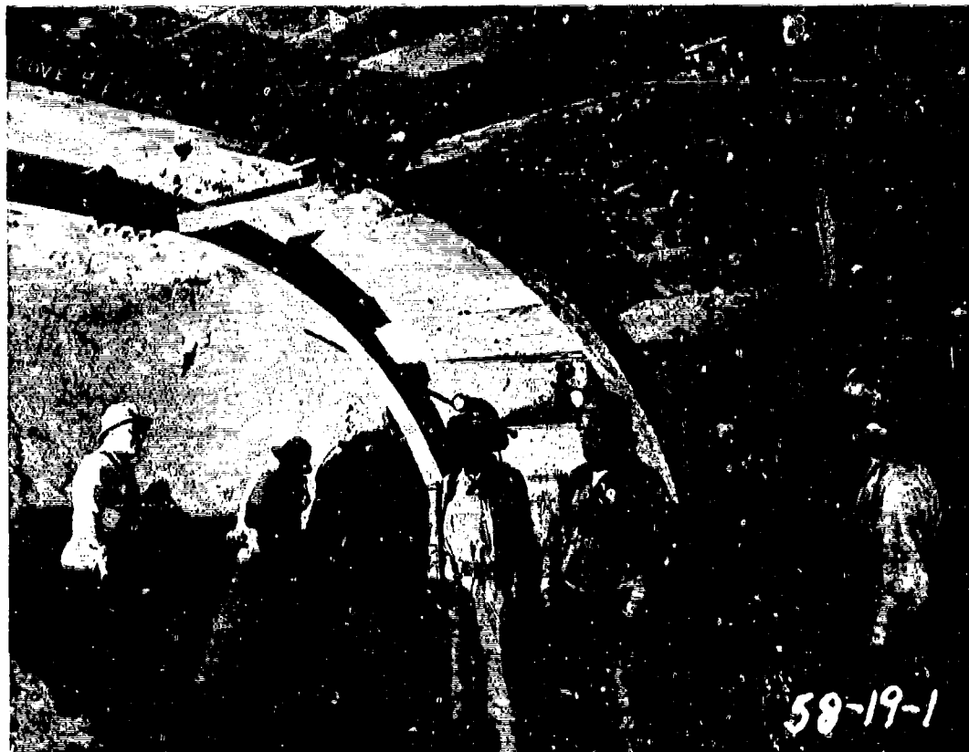
Figure No. 5. Steel Supports in No. 1 Alcove — Side Drift U-12b.03
