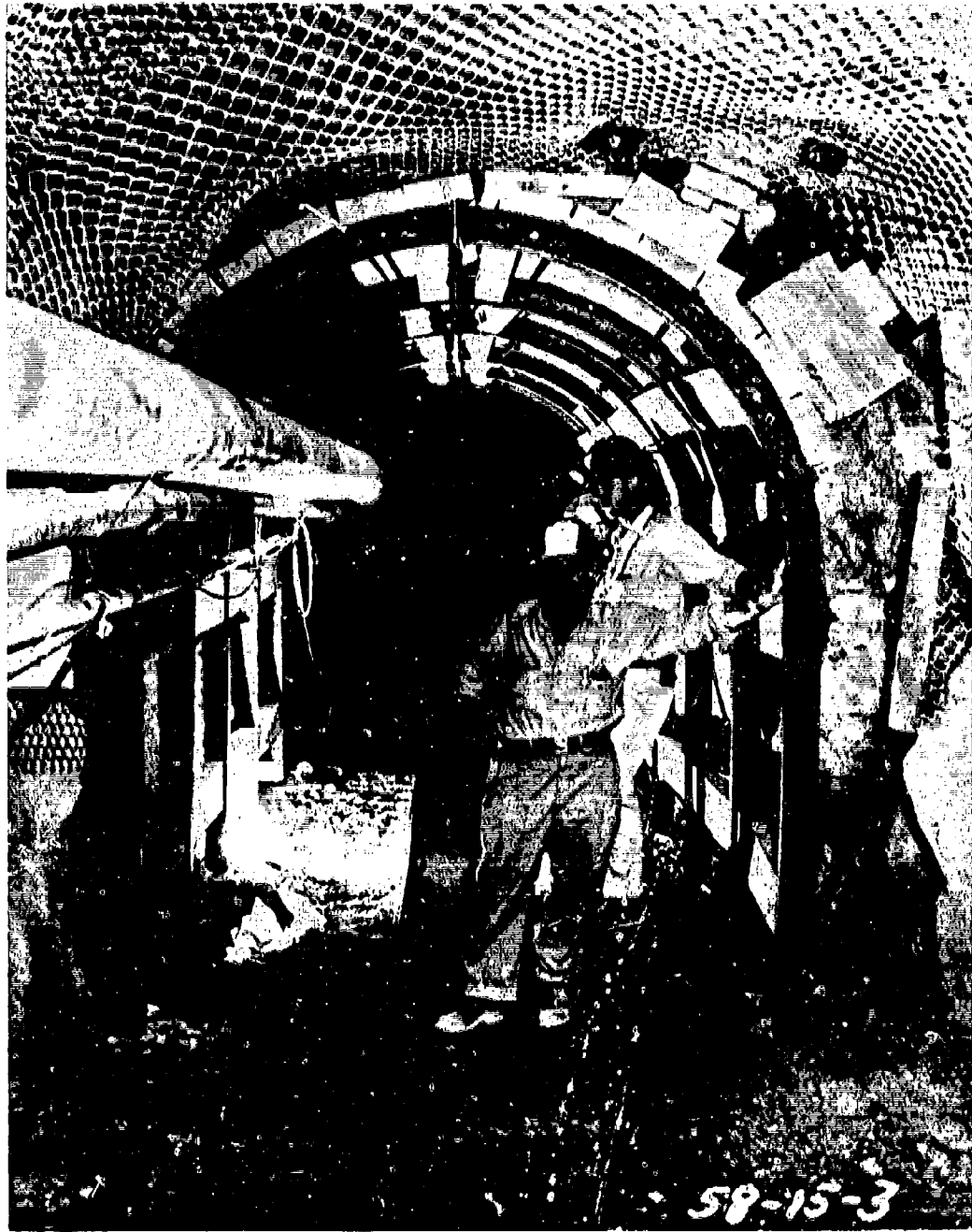
Figure No. 21. Transition from Wire Mesh to Steel Supports in Side Drift U-12b.04
