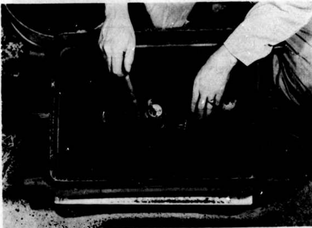
Figure 80. Ramming a deep pocket.
