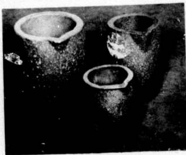
Figure 188. Lip-pouring crucibles.
