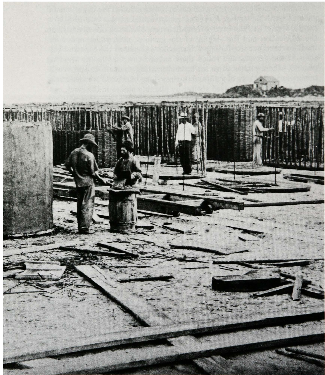
Fabrication of gabions. Workmen at right set stakes in wooden bottoms as man to their left performs "basket-weaving" function. Gabion in left foreground is covered with hydraulic cement. Old fort appears in background.
