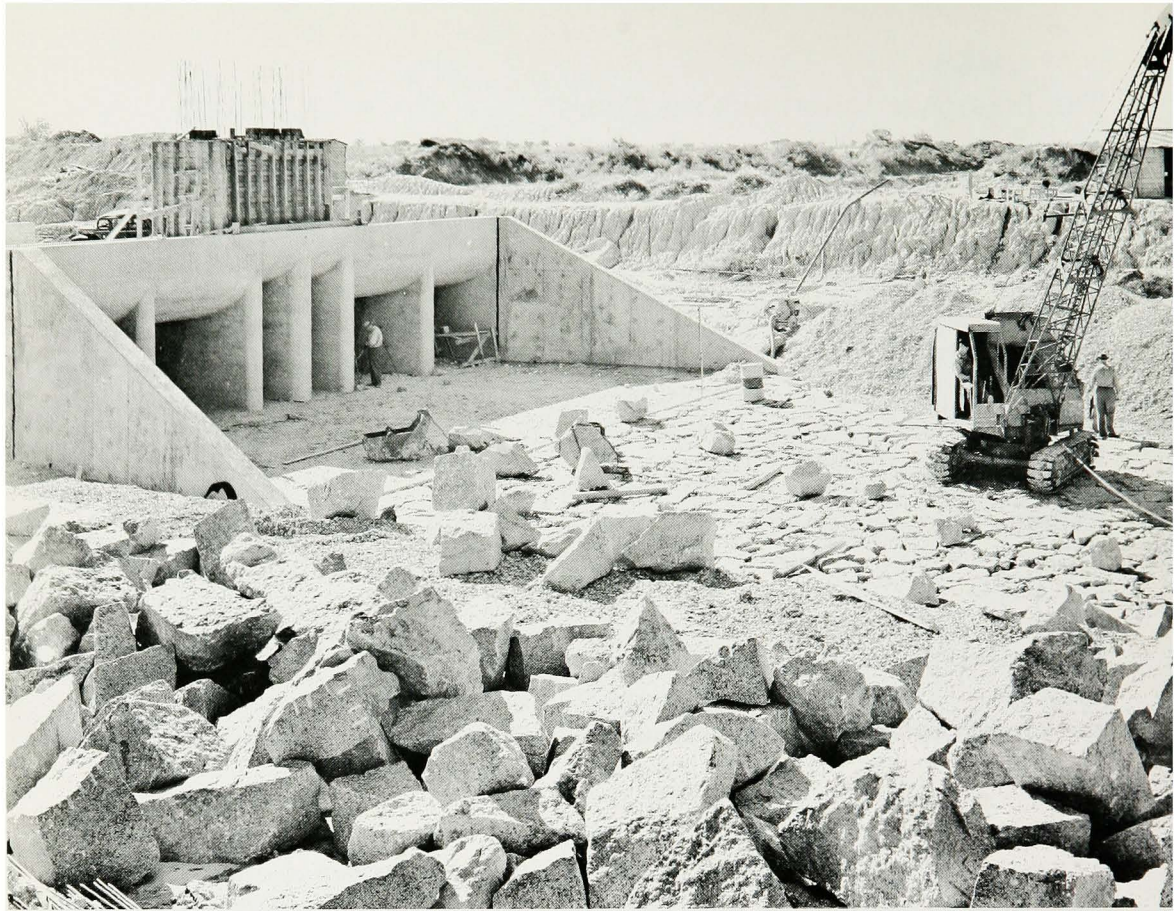
Barker Dam construction. Placing riprap at upstream end of outlet works, September 23, 1942
