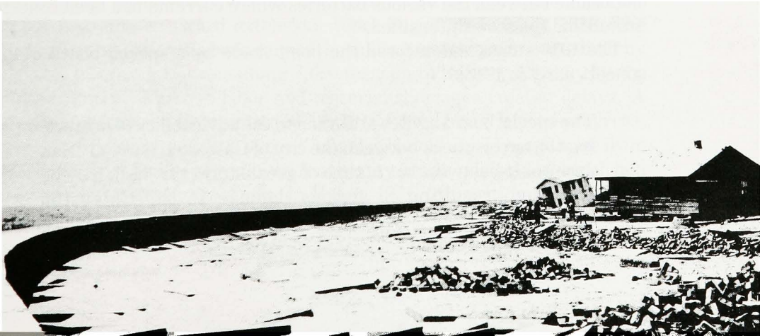
Damage to seawall embankment at Sixth Street from 1915 storm
