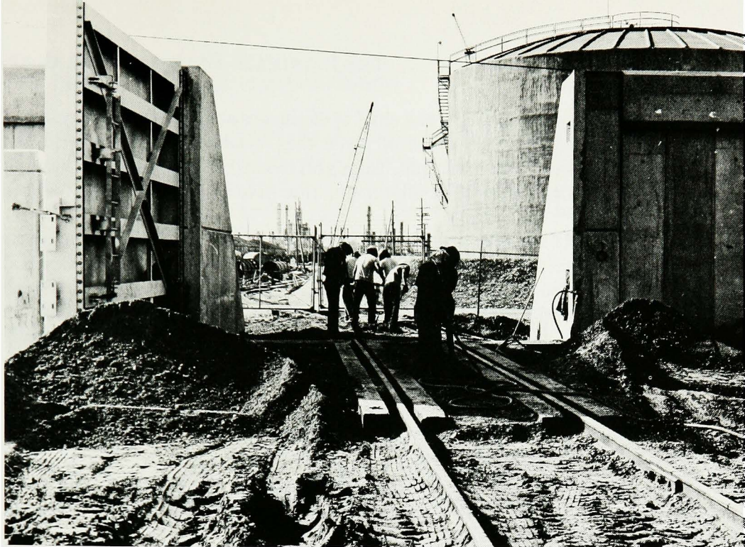
Workmen at railroad opening of closure structure in Texas City flood-wall, 1975
