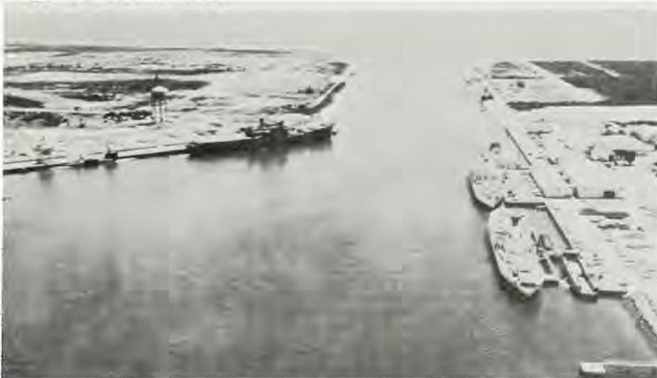
*Man-made Port Canaveral, built under Corps of Engineer contracts and supervision in 1950-52, has since undergone frequent modifications in depth and facilities. This 1967 view shows missile tracking ships in right center and Navy's Observation Island test ship at left center. Courtesy Corps of Engineers.*
