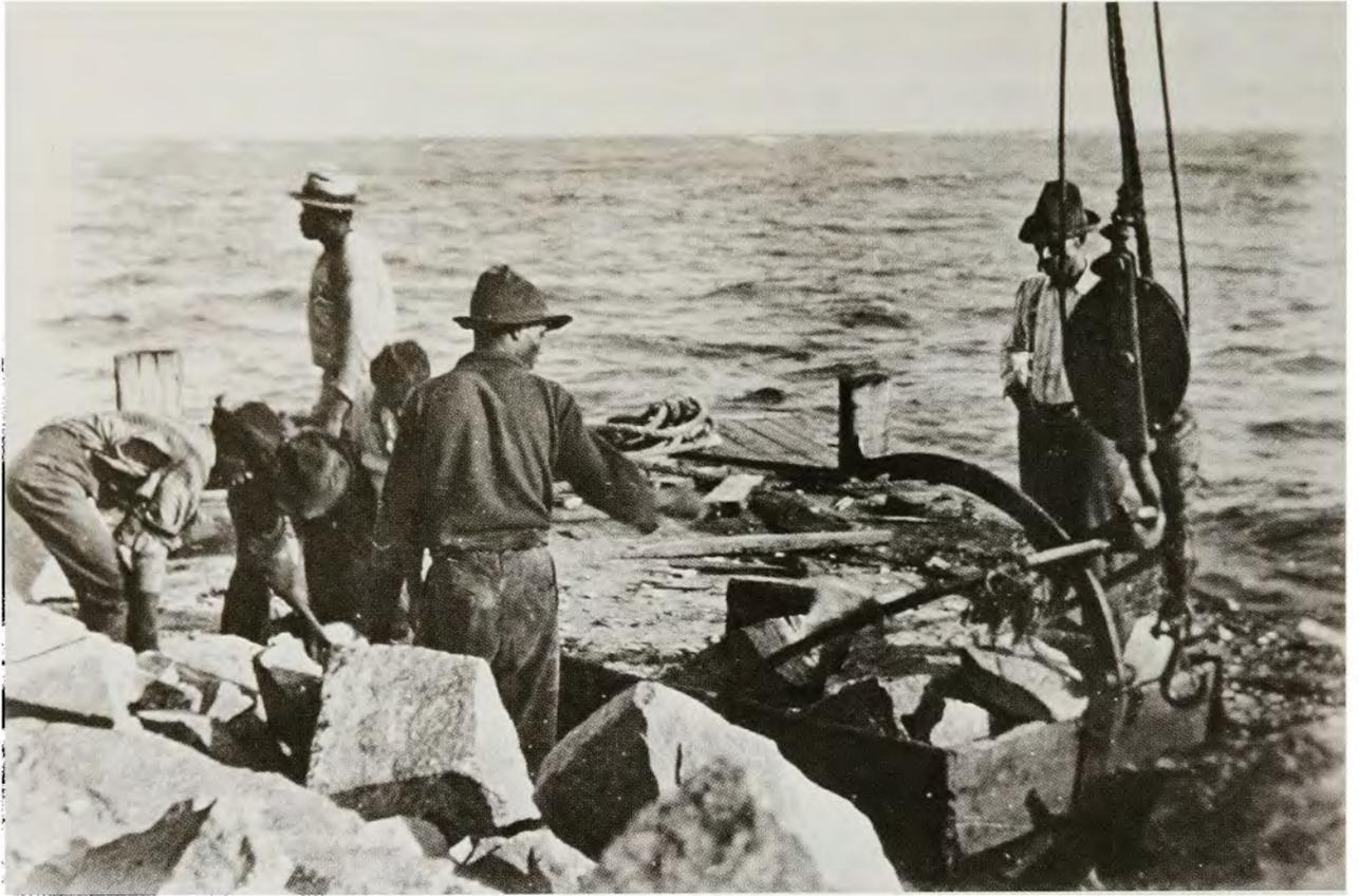
*Workmen unload small pieces of stone onto jetty in 1900 (top). Another load of stone arrives for the jetties (bottom).*
