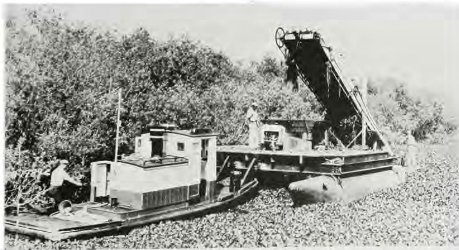
*Conveyor system pulls Hyacinths into shredder on Lake Okeechobee, March 1973 when Corps of Engineers conducted crash spraying program. Courtesy Corps of Engineers.*
