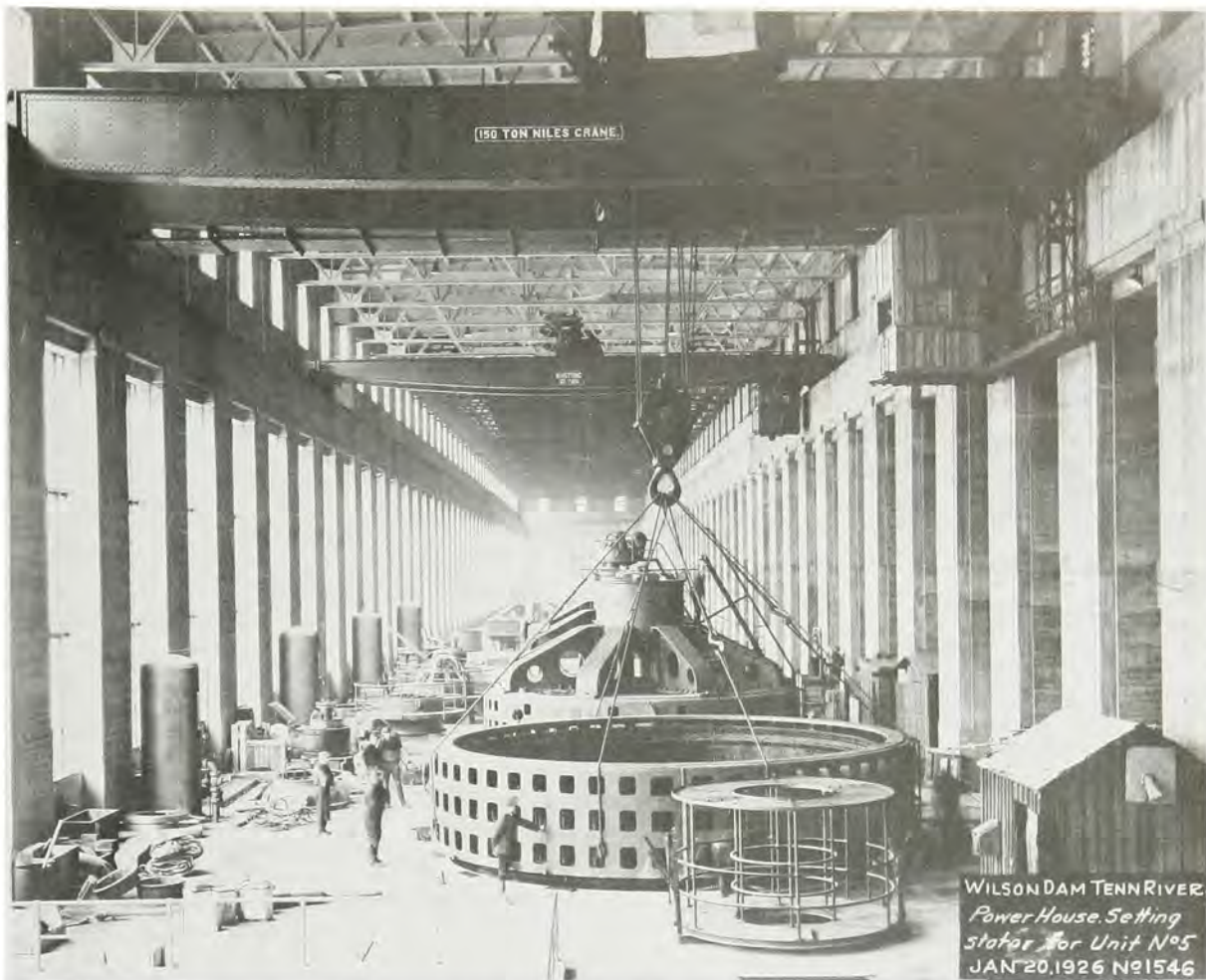
Installing the Wilson Dam power generators, 1926.
