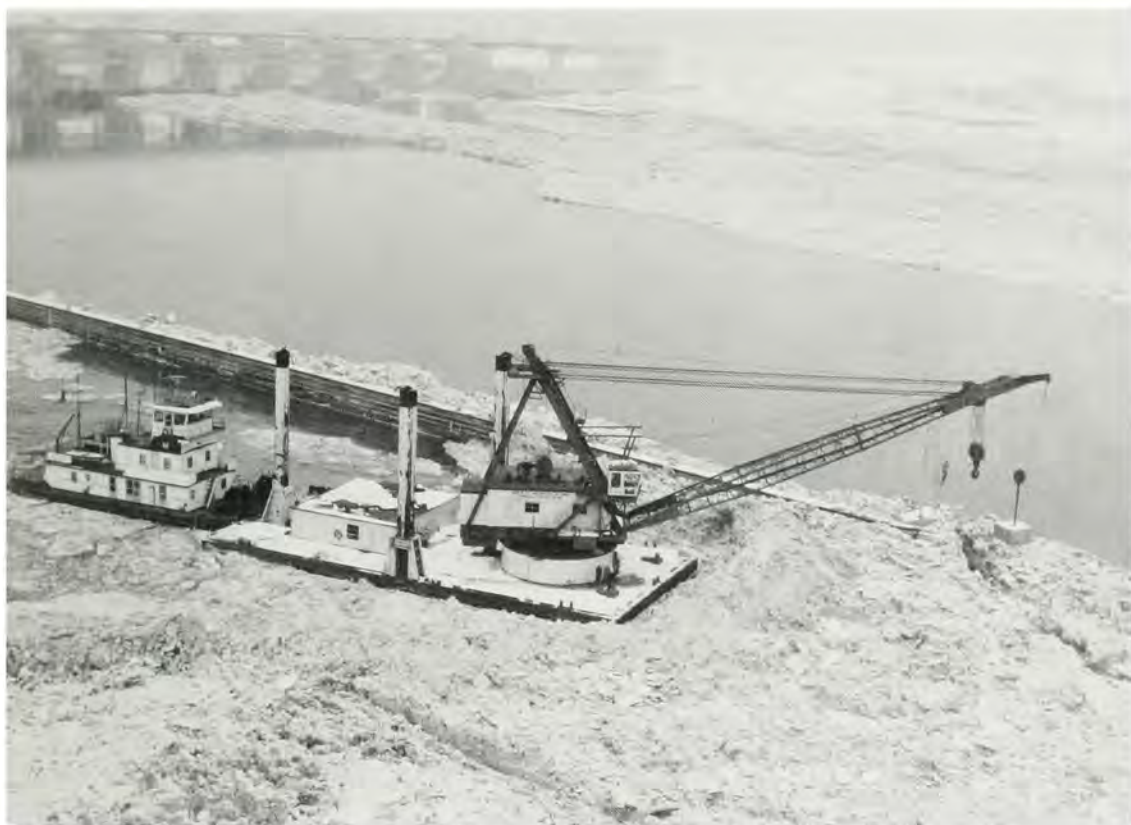
District towboat and derrickboat breaking ice at the entrance to Markland Locks, February 3, 1978.
