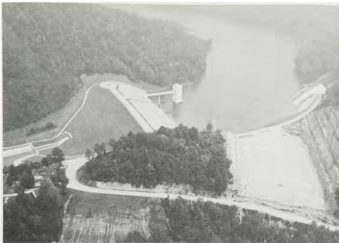
Aerial view of Carr Fork Dam and Lake near Hazard, Kentucky. The dam and control tower are in the center of the picture, the outlet and stilling basin on the left, the spillway cut into the rock at the lower right, and a boat launching ramp at right center.
