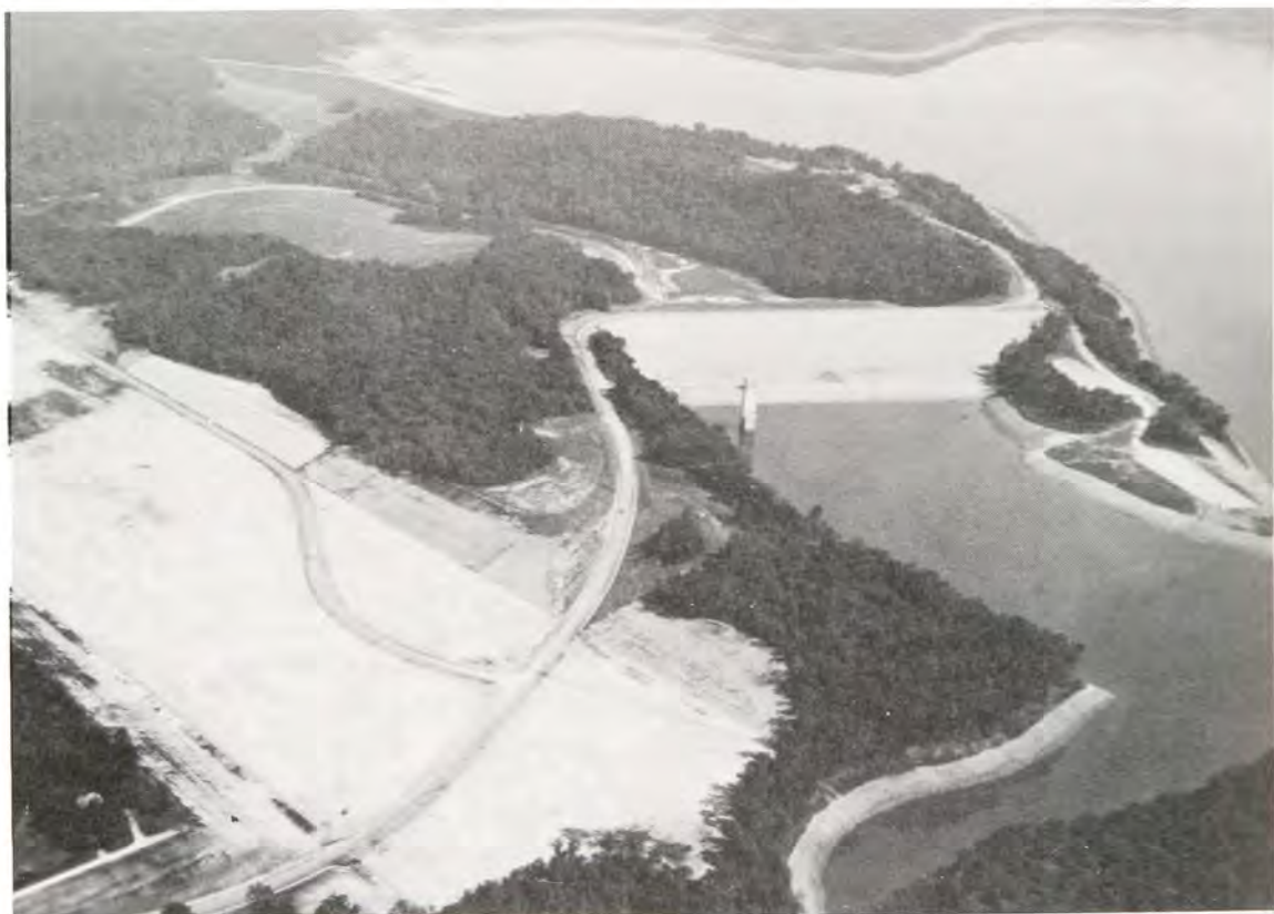
Aerial view of East Fork (William H. Harsha) Dam and Lake, September 28, 1979. The light-colored rectangle on the left is the huge spillway where the rock removed was placed into the dam. A large saddle dam is visible near the top of the picture.
