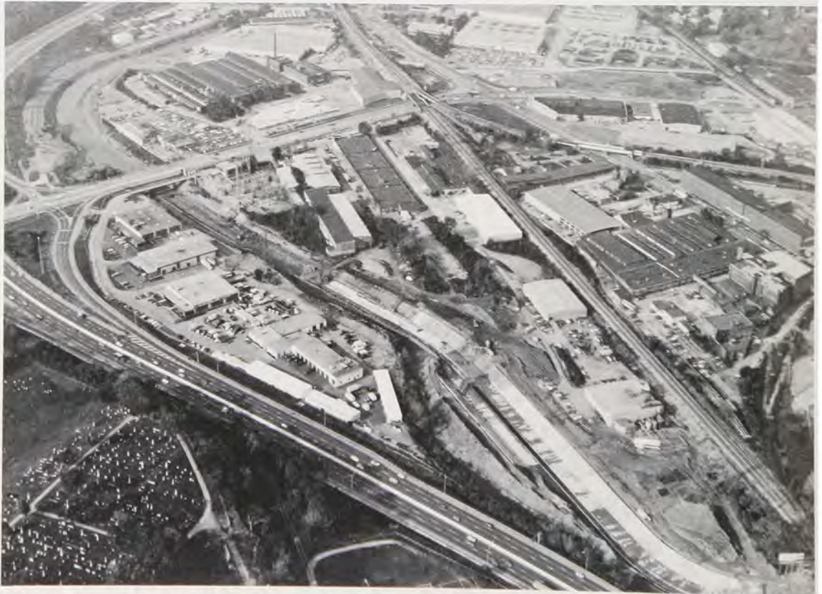
Aerial view of part of the Mill Creek local protection project, October 21, 1982. The new lined stream channel is visible amongst the industrial plants and paralleling the highway.
