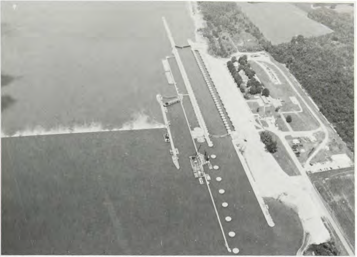
Lock and Dam 52 near Paducah, Kentucky, had a temporary 1200-foot lock added in 1969. In the picture the 600-foot lock is on the left with a boat entering it; the 1200-foot lock with the steel cell walls is at right next to the bank.
