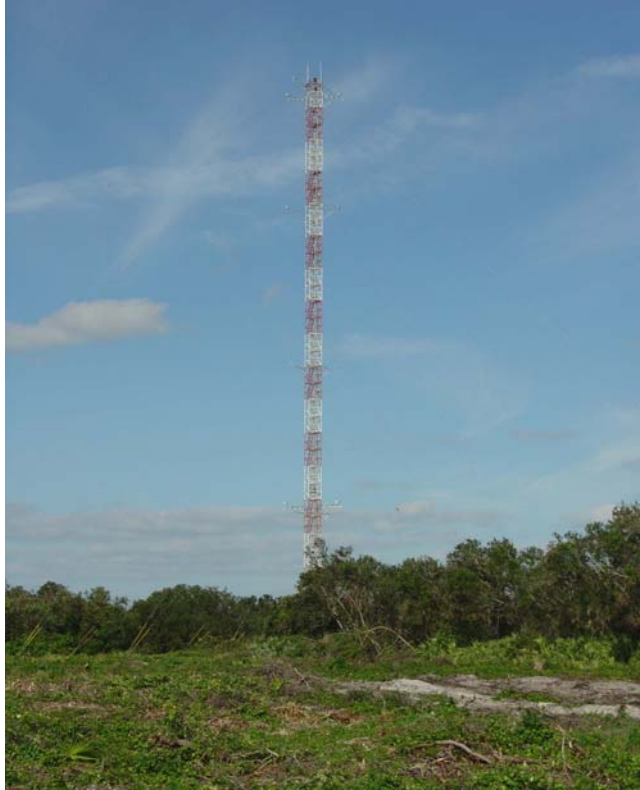
Figure 1-4: Example Communication Tower
