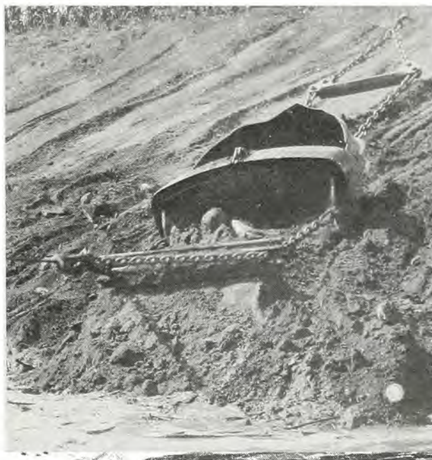
A grading bucket taking the slope down to proper incline for bank paving. Reelfoot Front, 1932.
