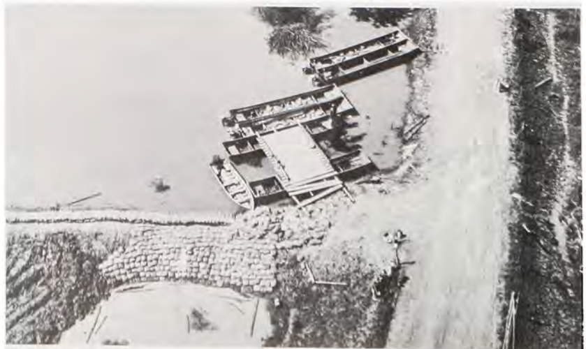
Emergency dock construction as used during floodwater. Filled sacks are trucked to dock, loaded into pontoons, then taken to endangered sites. Note also sandbag plug in levee breach. May 29, 1943, Booth's Point.
