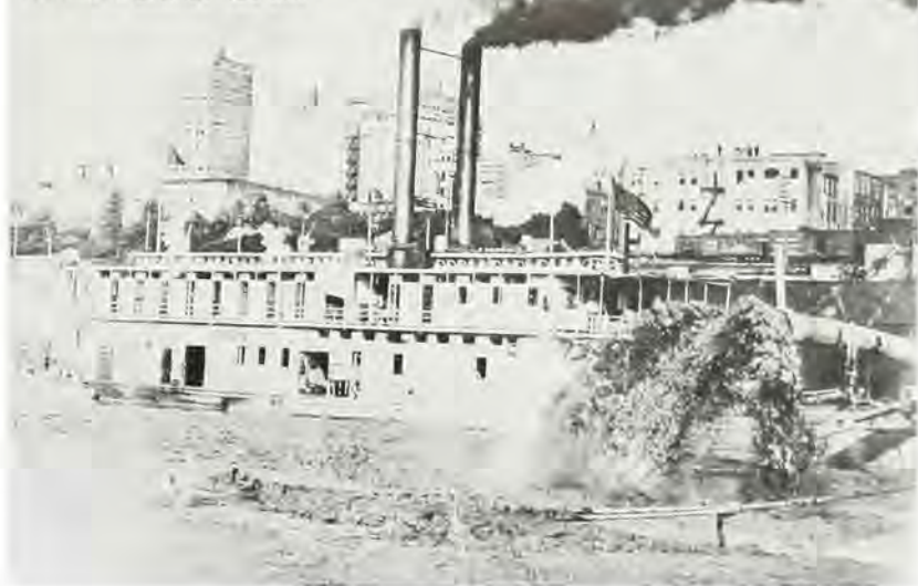
MISSISSIPPI RIVER DREDGING DISTRICT DREDGE "EPSILON" IN MEMPHIS HARBOR 32 INCH PIPE LINE DREDGE NO PROPELLING ENGINES - BUILT IN 1898 LENGTH 157 FT. BEAM 40 FT. DEPTH 7 FT. 6 IN. DRAFT 46 IN. TWO HORIZONTAL TANDEM COMPOUND NON-CONDENSING MAIN PUMP ENGINES 750 I.H.P.
