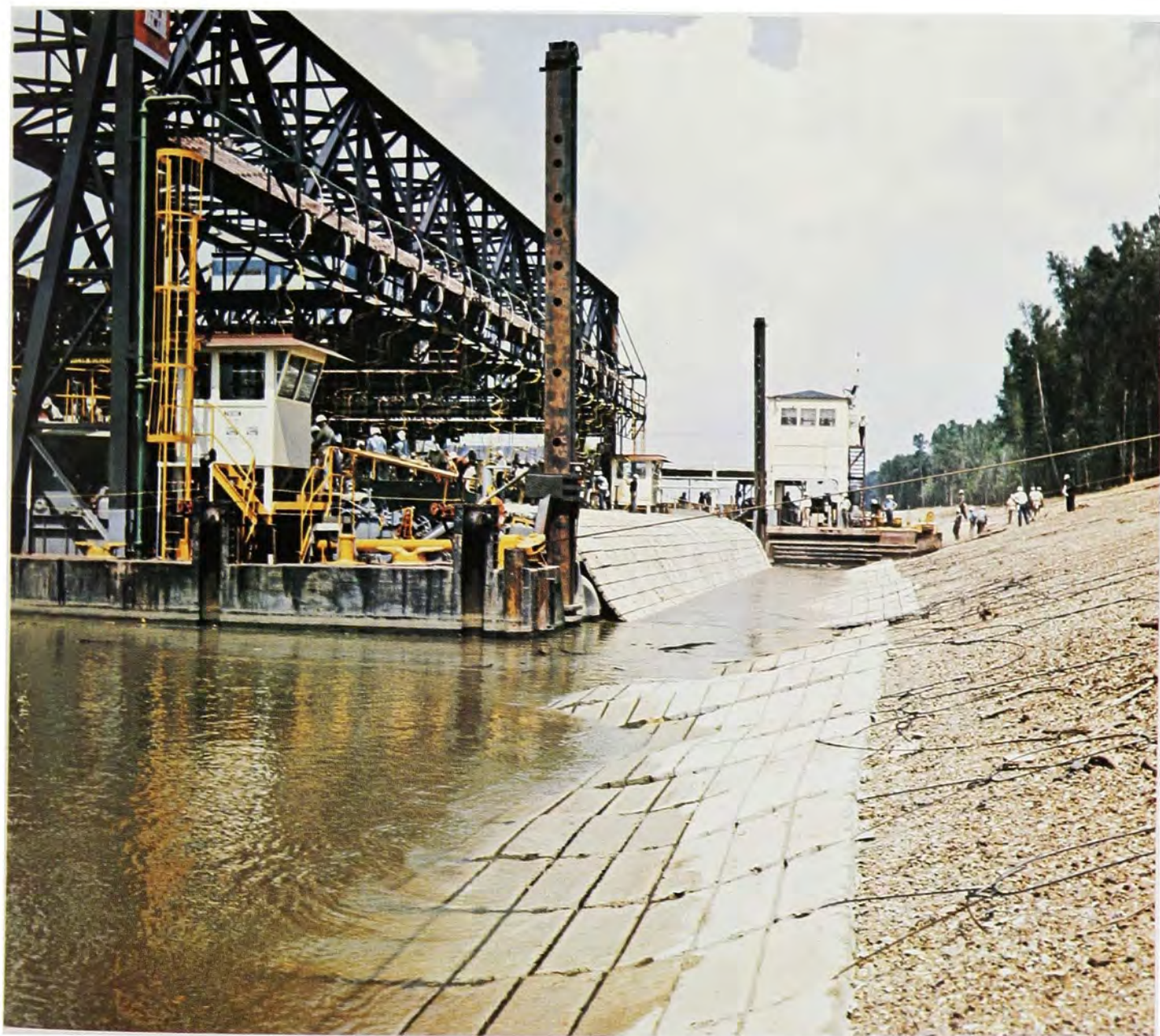
The Memphis District mat-laying plant at work. Though capable of greater output, the plant will average sinking about 330 squares per hour on a ten hour shift, or 330,000 square feet of articulated mat in a ten-hour work day.
