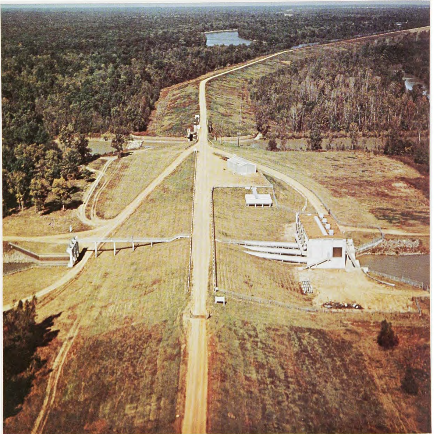
The Graham Burke Pumping Plant, in Phillips County, Arkansas, landward of the White River Backwater Levee. Named for the late Judge J. Graham Burke of Helena, the plant serves approximately 145,500 acres of alluvial lands by removing water impounded between the White River Levee and the Mississippi River levee system. A considerable portion of the sump area is part of the White River National Wildlife Refuge. The Plant was completed in November, 1964.
