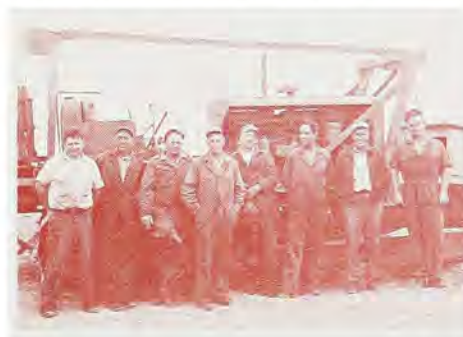
Debris collection crew – October 1946.
