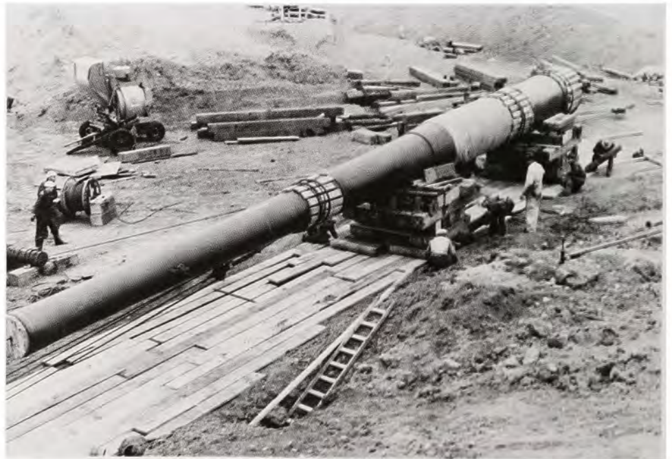
Moving the gun from one place to another required patience and careful placement of timbers and rollers.
