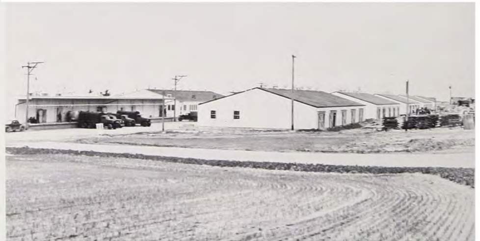
Storage facilities—Fort Ord—January, 1942.
