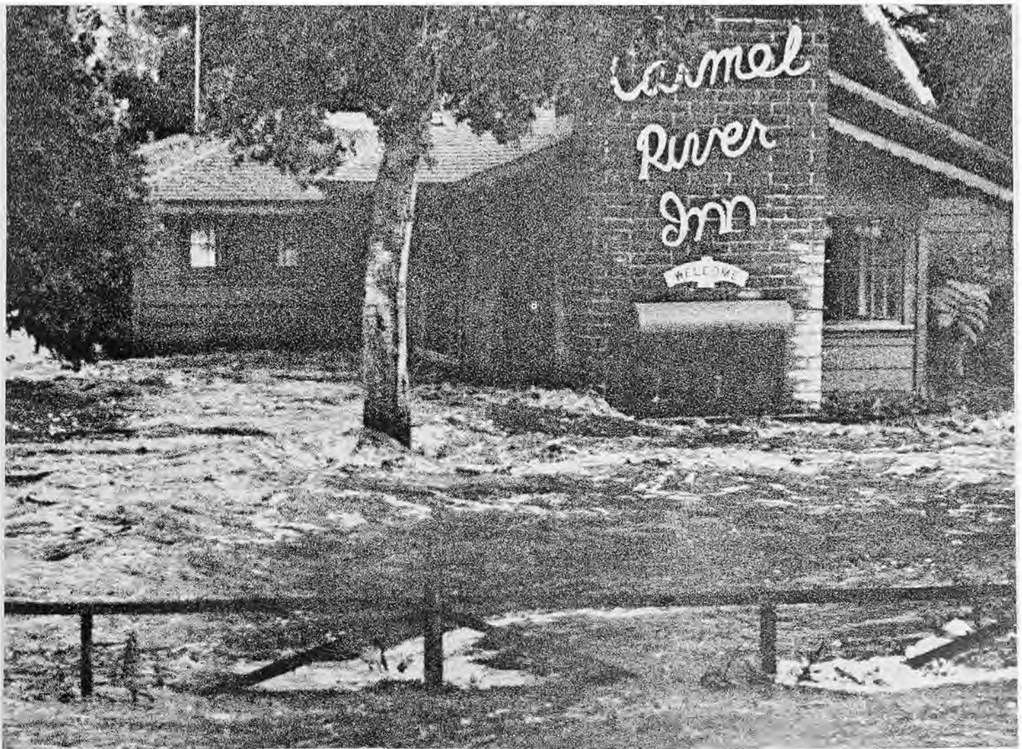
Carmel River—flooding the Carmel River Inn—1967.
