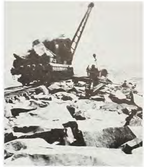
Placing stone on the breakwater – July 1921.
