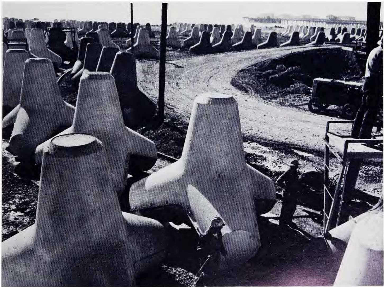
Tetrapods await placement at Crescent City – 1956.
