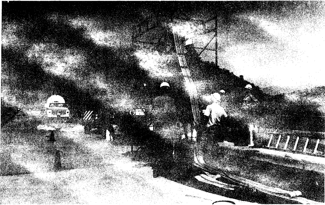
Figure 101. Approximately one-half of the liner tube installed, Pine Flat Dam
