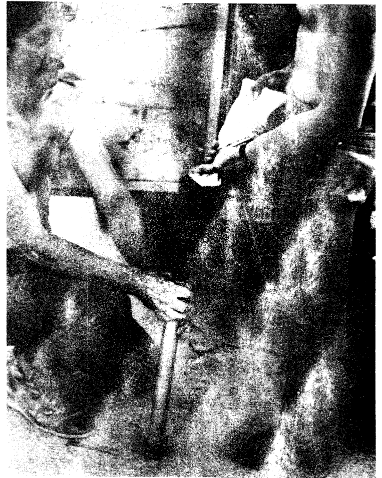
Figure 152. Steel pipe filled with lead shot to weight the composite sleeve, Bagnell Dam
