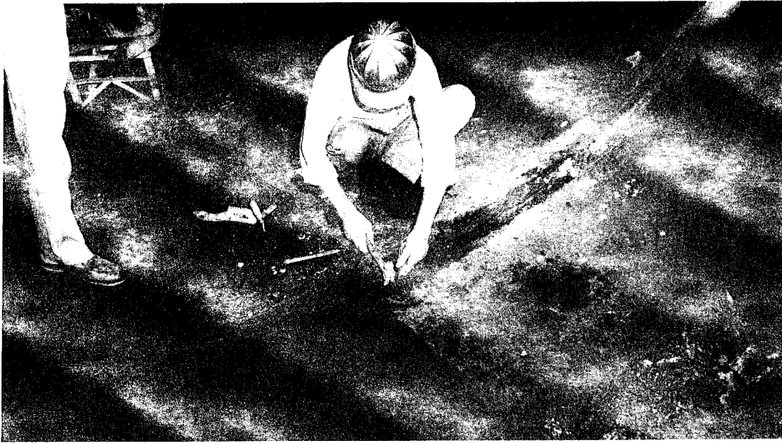
Figure 17. Removal of a portion of the remaining concrete key in preparation for repair, Sardis Dam
