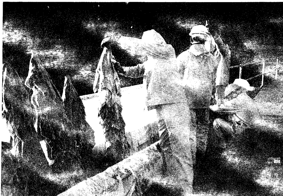
Figure 144. Soaking burlap "Christmas trees" in polyurethane foam grout, Easton Reservoir Dam
