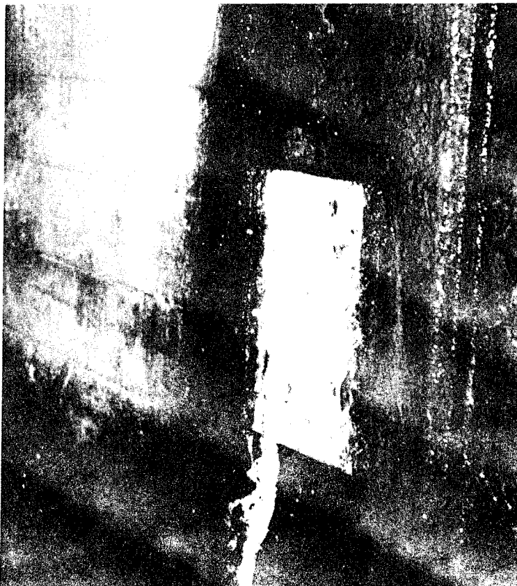
Figure 146. Leakage of joints 15 and 17 as seen in the gallery, Bagnell Dam
