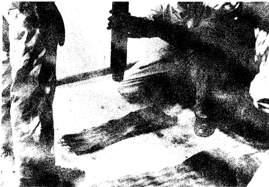
b. Saturated bag on top of drill hole awaiting insertion
