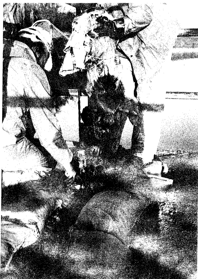
Figure 144. Soaking burlap "Christmas trees" in polyurethane foam grout, Easton Reservoir Dam
