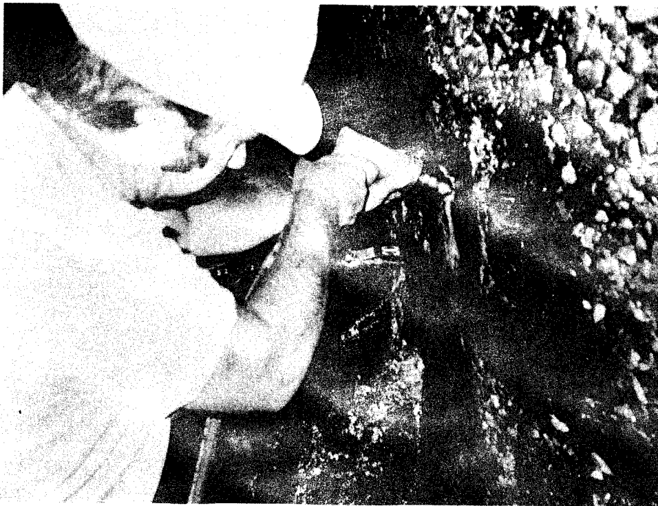
Figure 21. Drilling of injection port using pneumatic drill, Buckhorn Lake Dam, August 1986
