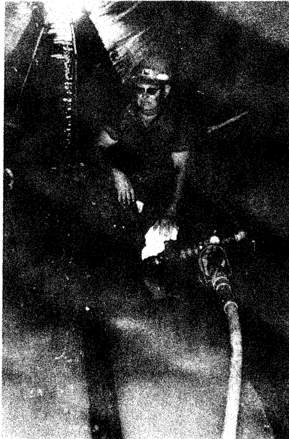
Figure 6. Control valve, Arkabutla Dam, 1977
