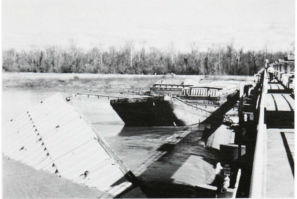
Barge accident, Wilbur D. Mills Dam, 1982
