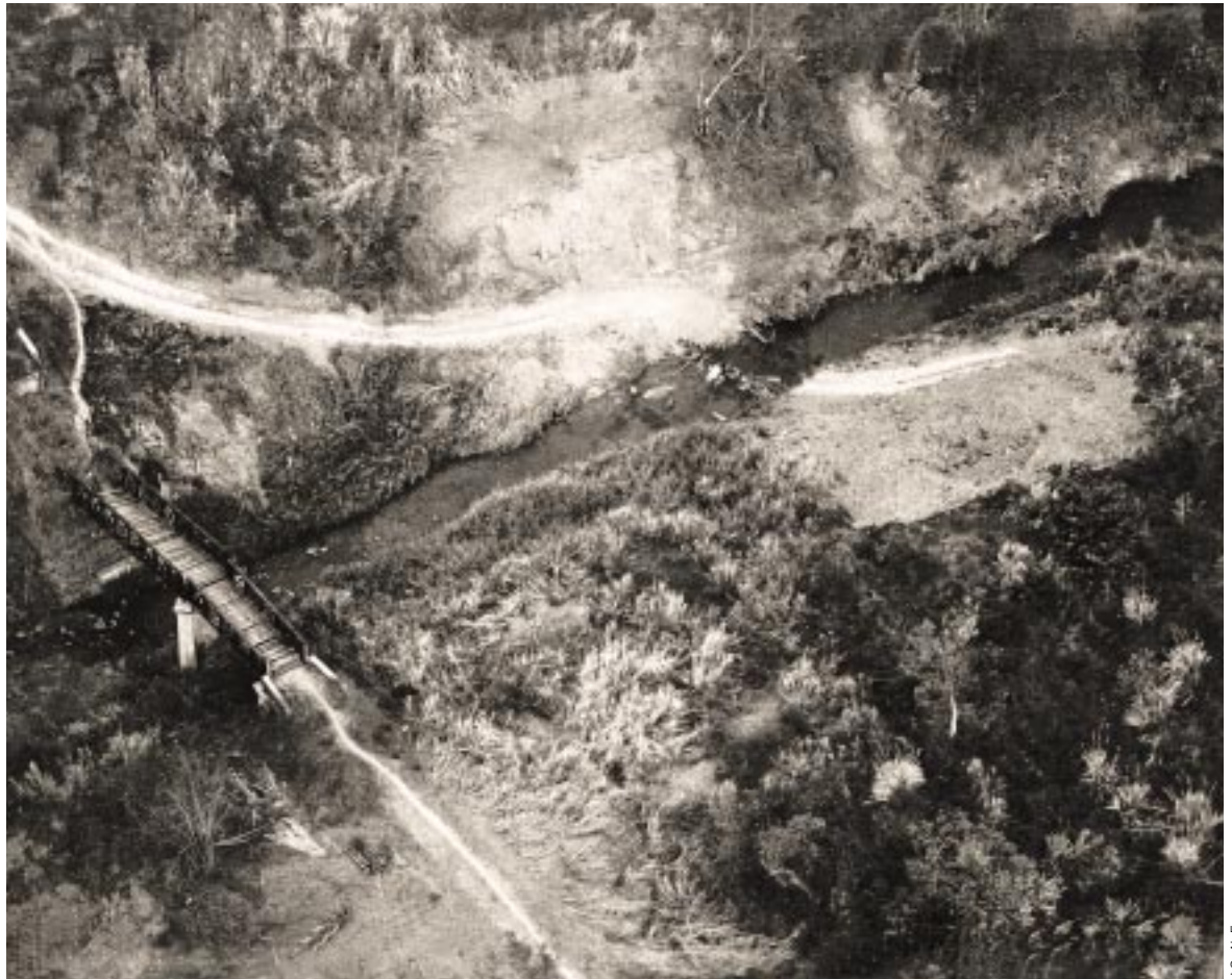
Typical ford bypassing colonial bridge on Route 9.
