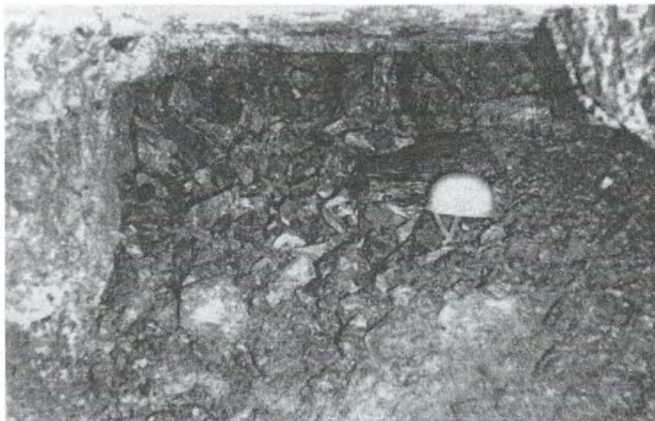
Figure 7.10: Photograph of loose rocks taken in adit #33 that crosses the cut-off screen as shown in Figure 5.6.
