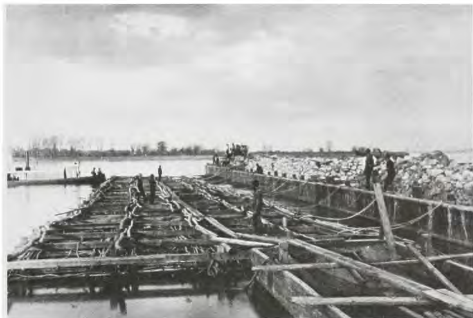
Mattress revetment is placed afloat prior to sinking under the weight of large stones.
