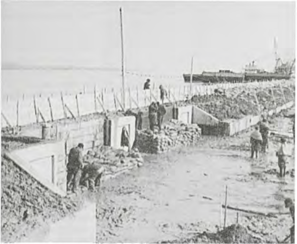
Raising the level of protection at Cairo during the 1937 flood.
