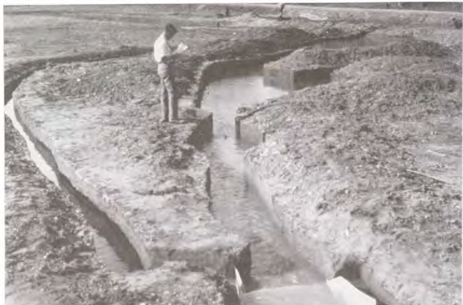
The Illinois River backwater model was the first outdoor model constructed at the Waterways Experiment Station.
