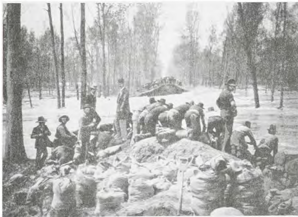
Tying the ends of a levee to prevent further collapse.
