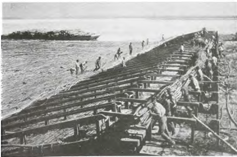
Weaving willow mattress revetment. MRC operations such as these did not curtail operations of the Corps of Engineers.
