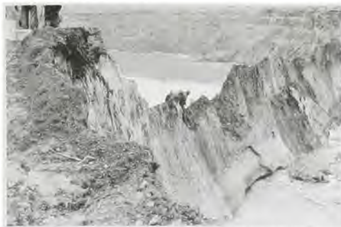
An earth plug is all that separates the two pilot channels. Note the difference in the water elevations of the upstream and downstream pilot channels.
