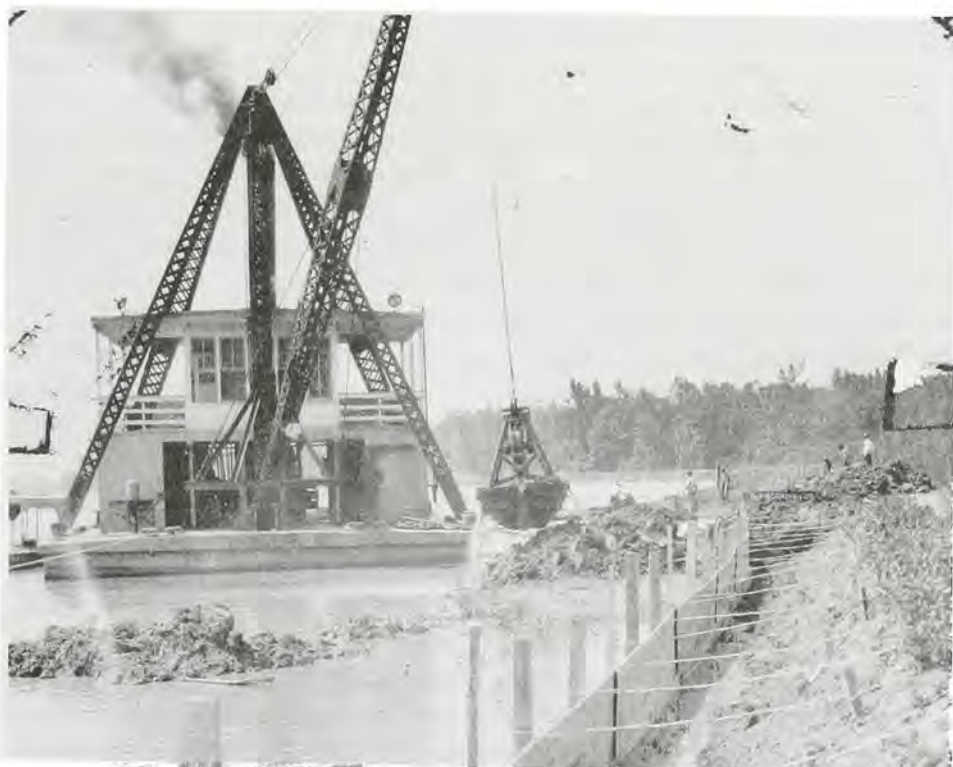
Protecting the riverside slope of a levee during the 1929 flood.
