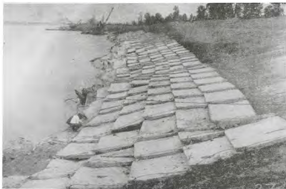
Lapped slab revetment.
