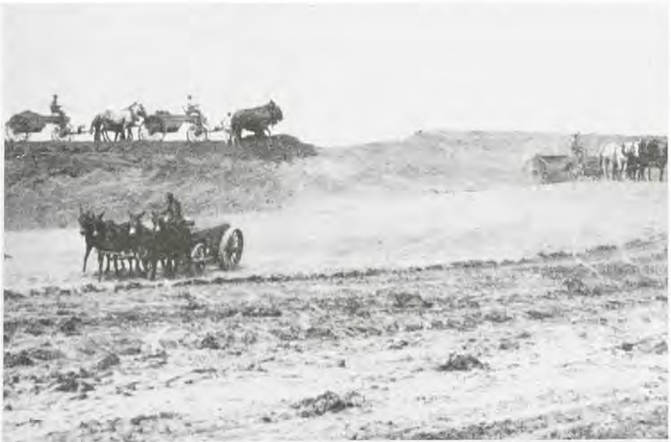
Mules and wagons are used to construct levees in the St. Francis Levee District in 1909.
