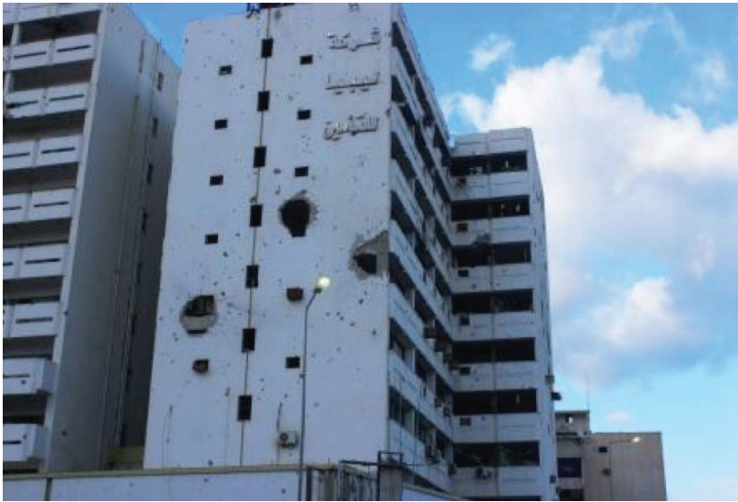
Figure 3.3 The Tamin Building, Tripoli Street, Misrata
