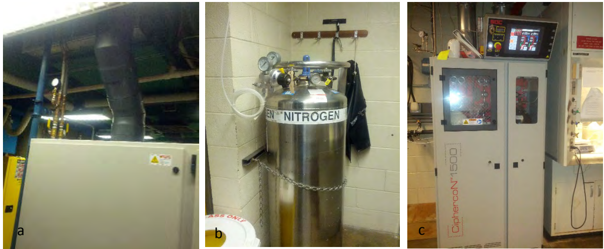
Figure 2 (a) Installation of exhaust system to the reactor and the rest of the fit up equipment (b) Installation of dedicated nitrogen for glove box and reactor purging (c) Installation of toxic gas cabinet for gases such as germane and 500ppm arsine in hydrogen.
