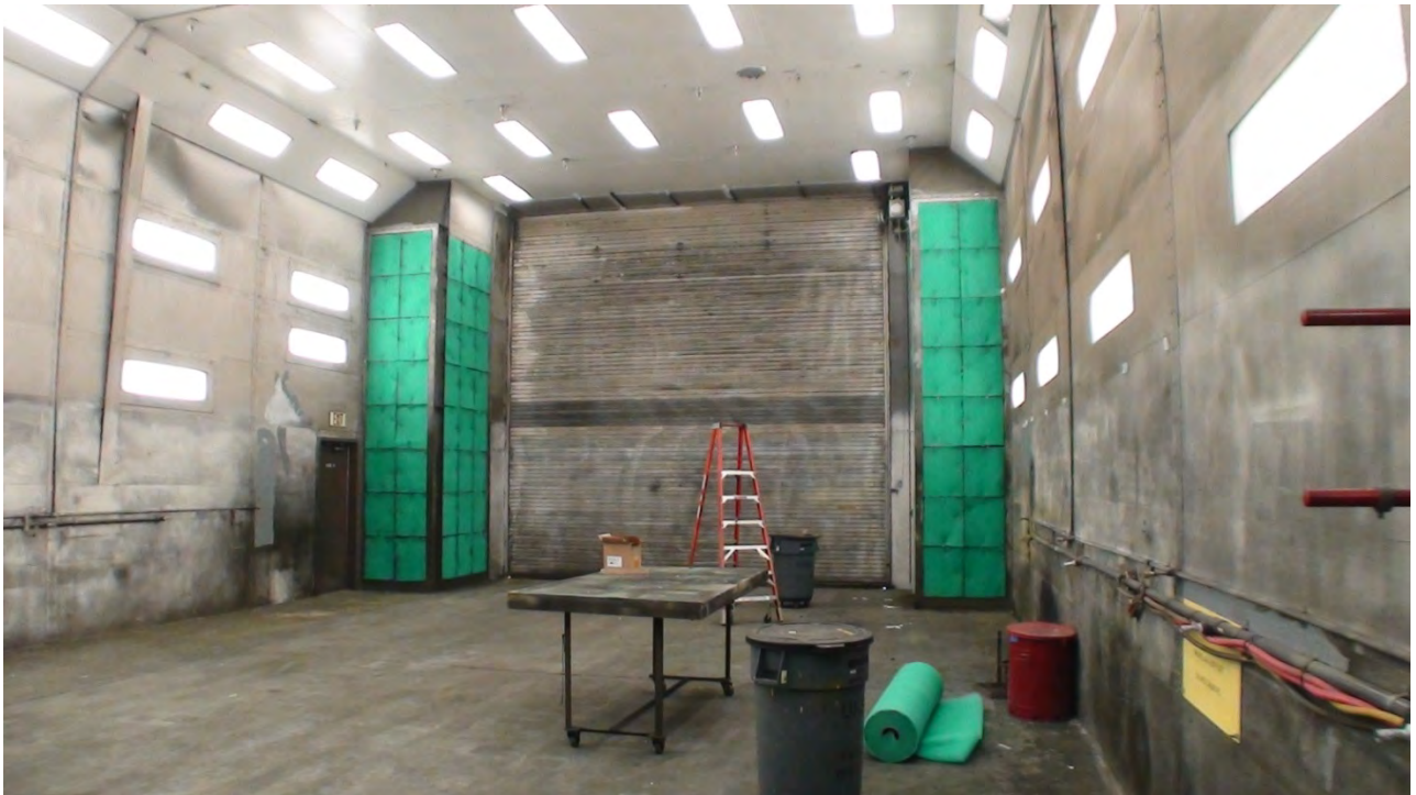
Figure 11: The Fort Lewis helicopter painting hangar. The exhaust filter columns can be seen on either side of the hangar door.
