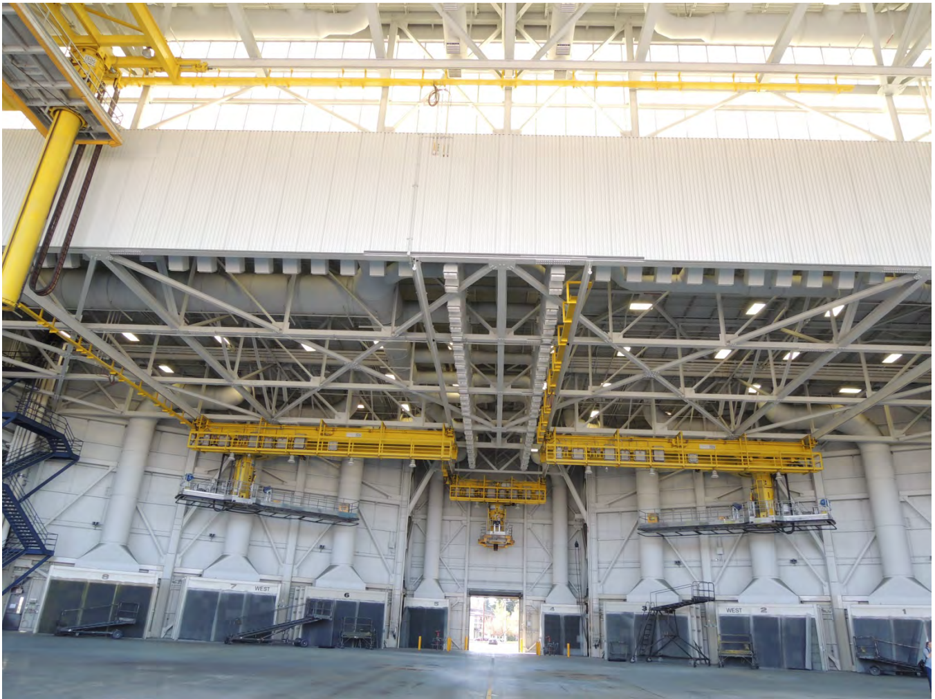
Figure 10: Photo of the JBLM corrosion control hangar. The eight large exhaust hoods are visible along the back wall, and the arrays of small square supply inlets can be seen on the ceiling.
