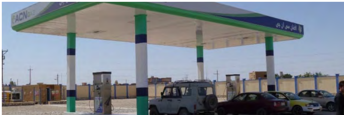
Figure 1 - The pumps at the CNG filling station constructed by TFBSO. Source: Central Asia Development Group
