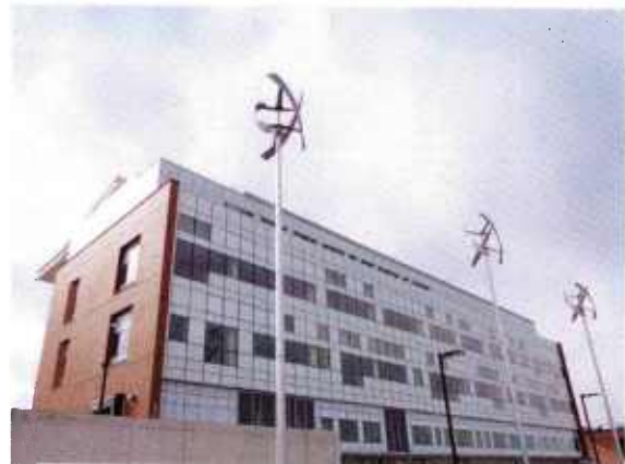
New GIS headquarters building
