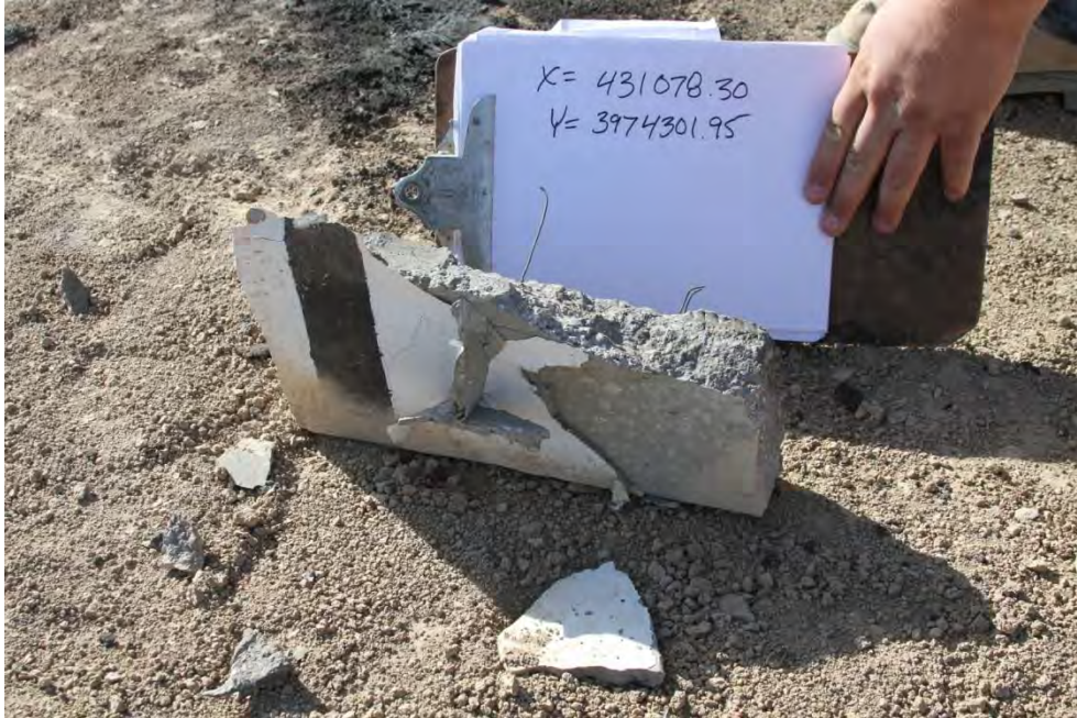
FIGURE V-G-4. Fragment From Front Wall Weighing 8,750 g and Found 17.5 m From Center of Original Structure (Test 4).
