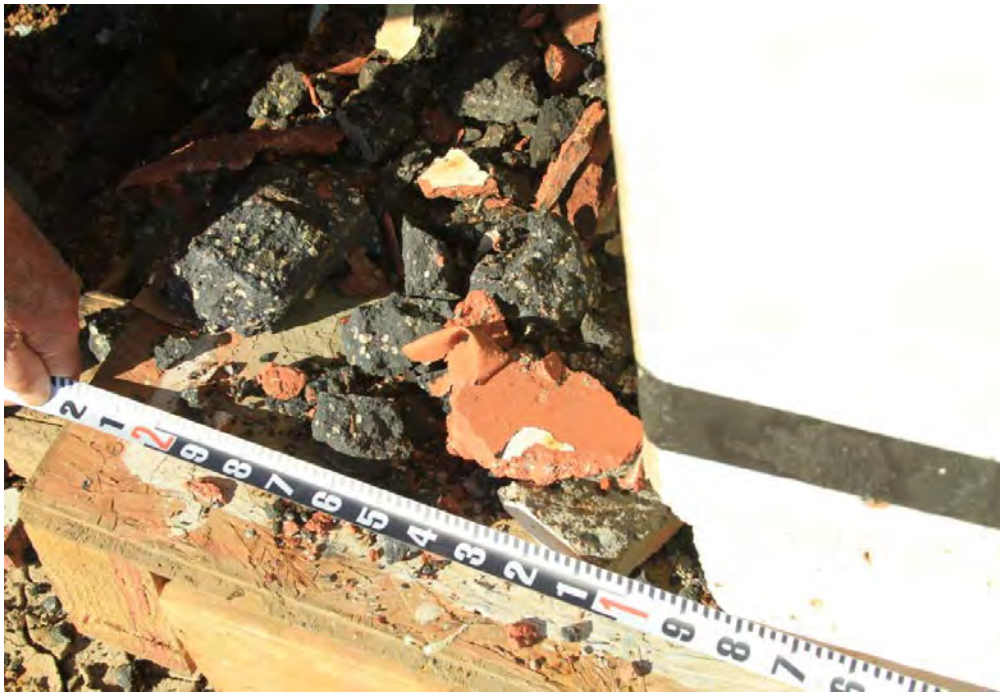
FIGURE III-28. East Wall/South Wall Intersection Displaced North by Almost a Foot From its Original Position on Pallet (Test 2).
