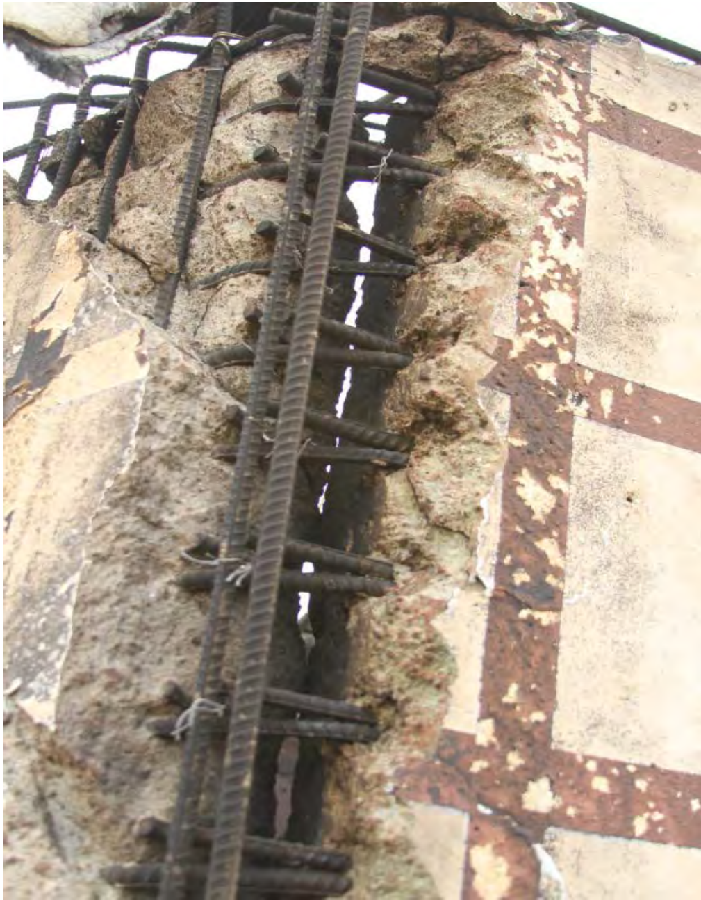
FIGURE III-25. Upper Portion of Western Wall/Northern Wall Intersection (Test 2).
