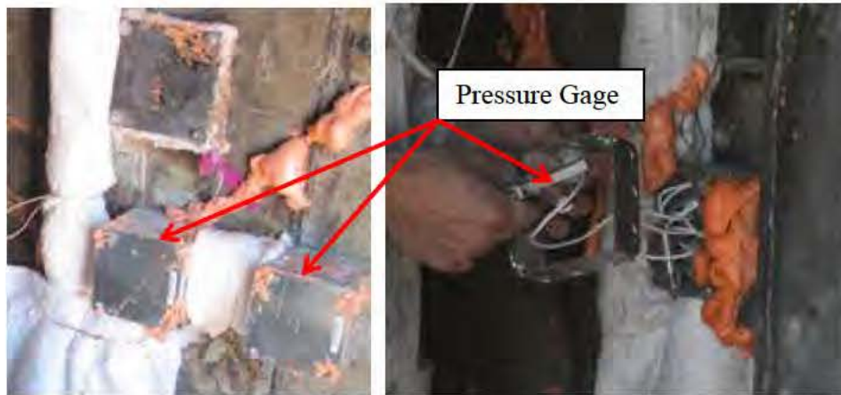
FIGURE I-9. Pressure Gage Mounted Inside Structure.
