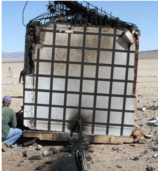
FIGURE V-29. West Wall Post Test (Test 4).
