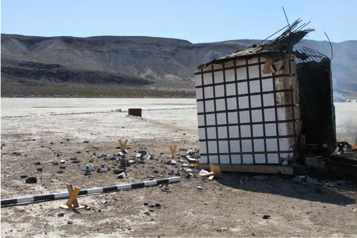
FIGURE V-26. East and North Walls Post-Test Structure (Test 4).
