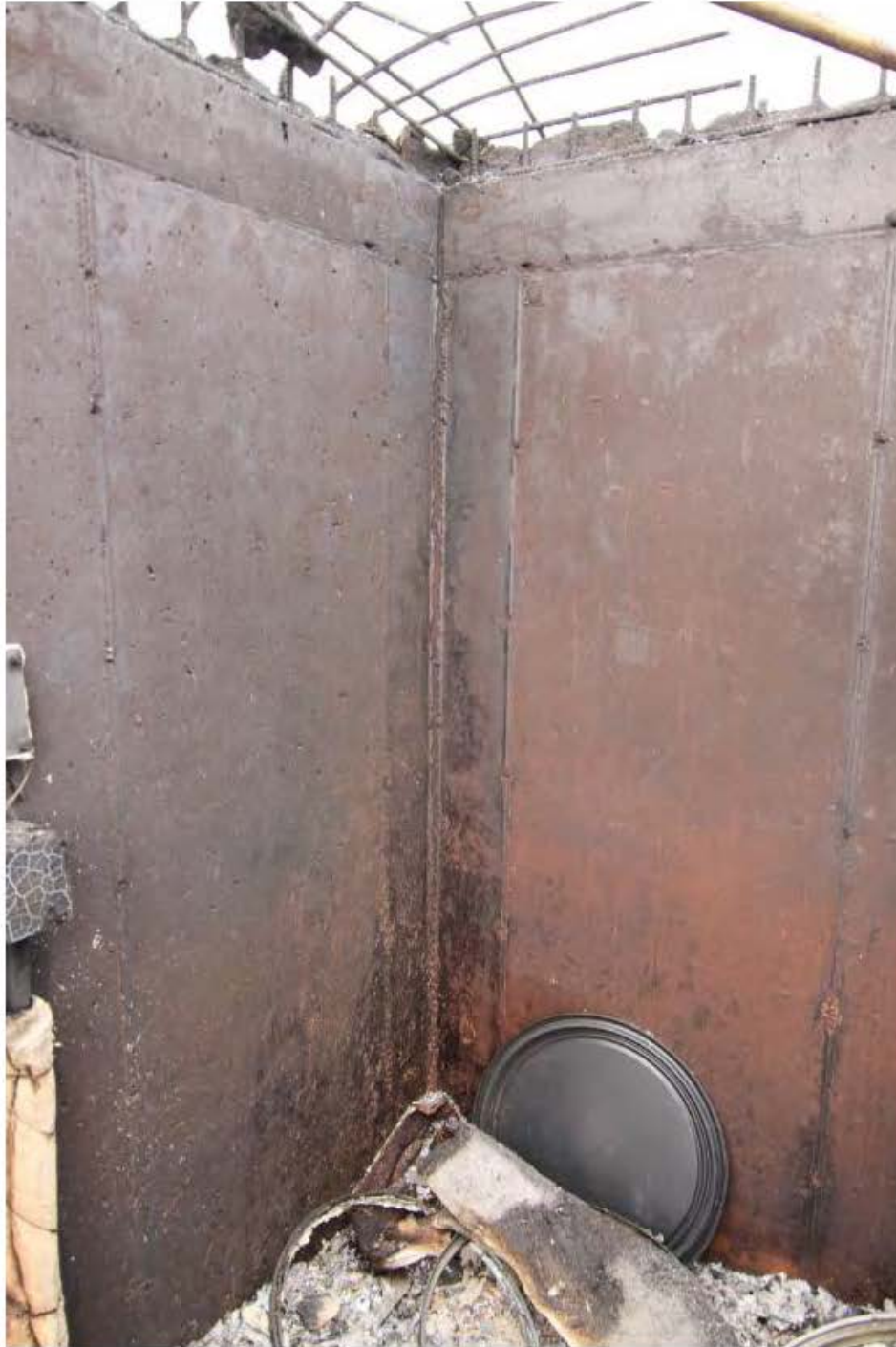
FIGURE III-13. Intersection of South Wall (Right) and East Wall (Left) (Test 2).
