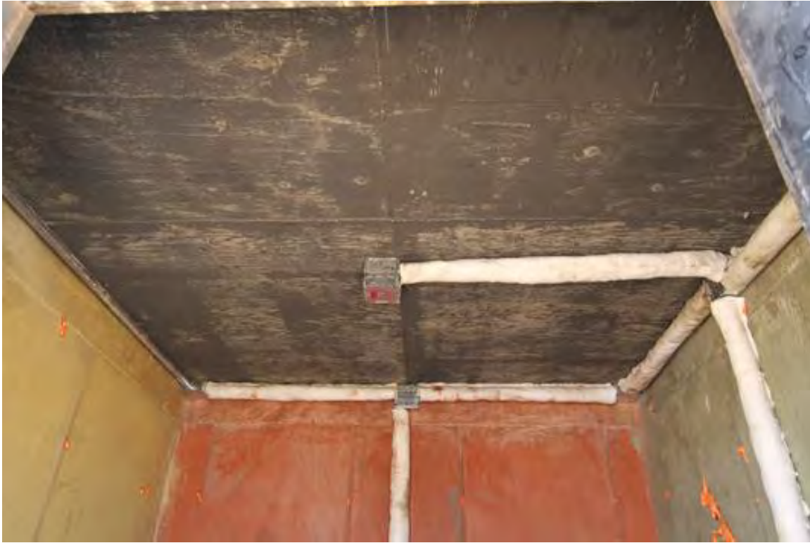
FIGURE I-8. Color Coded Concrete Walls. Black = roof, red = south wall, yellow = east wall, and green = west wall.
