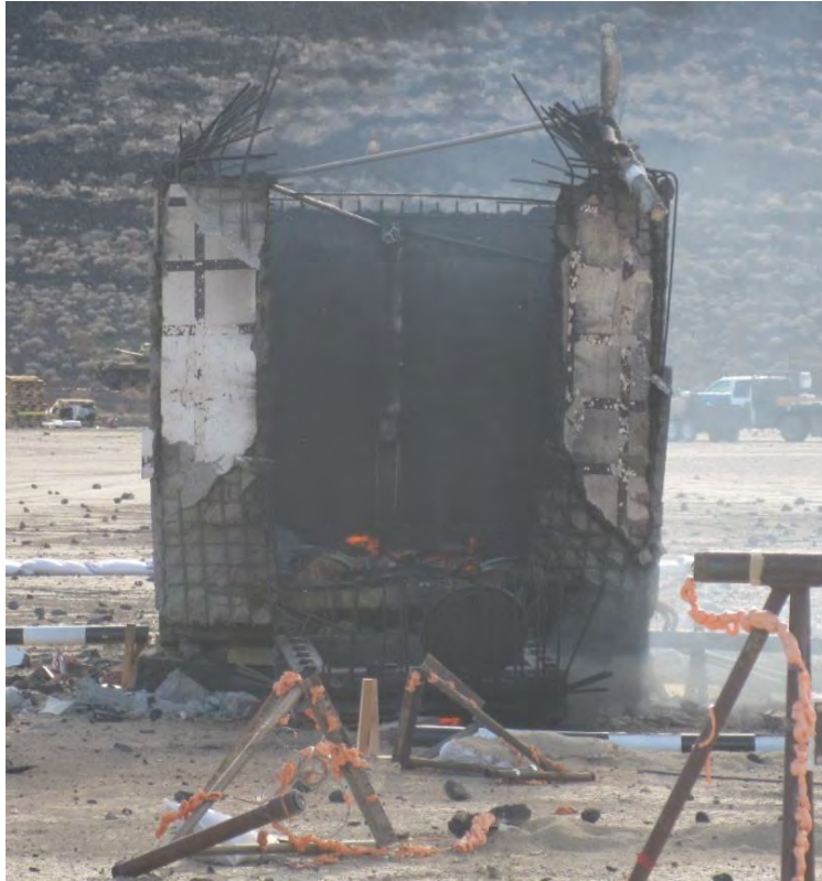
FIGURE VI-3. Test 2 Structure Post Test.
