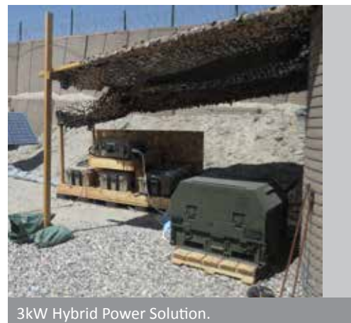
3kW Hybrid Power Solution.
