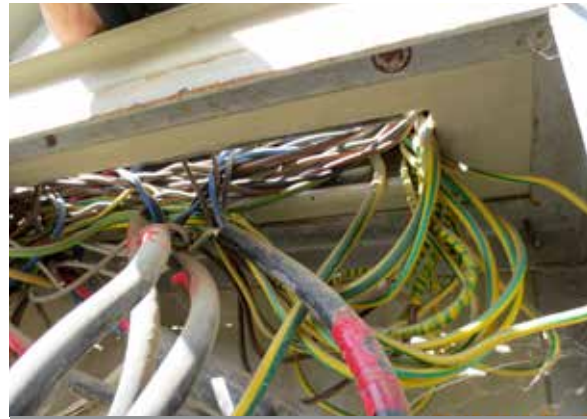
Improper electrical wiring at ODA Shinwar.
