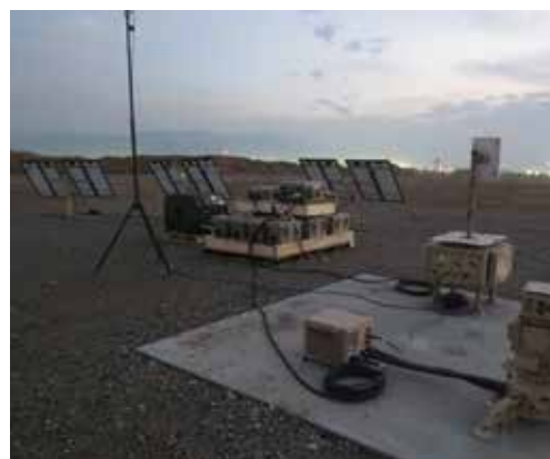
3kW Hybrid Power Solution.
