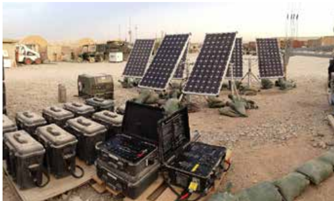
3kW Hybrid Energy System at FOB Pasab, Solar Stik 360
