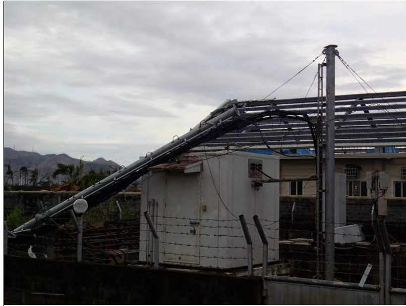
Figure 28. Broken Broadcast Tower Assessed by RTAT in the Aftermath of Typhoon Haiyan
