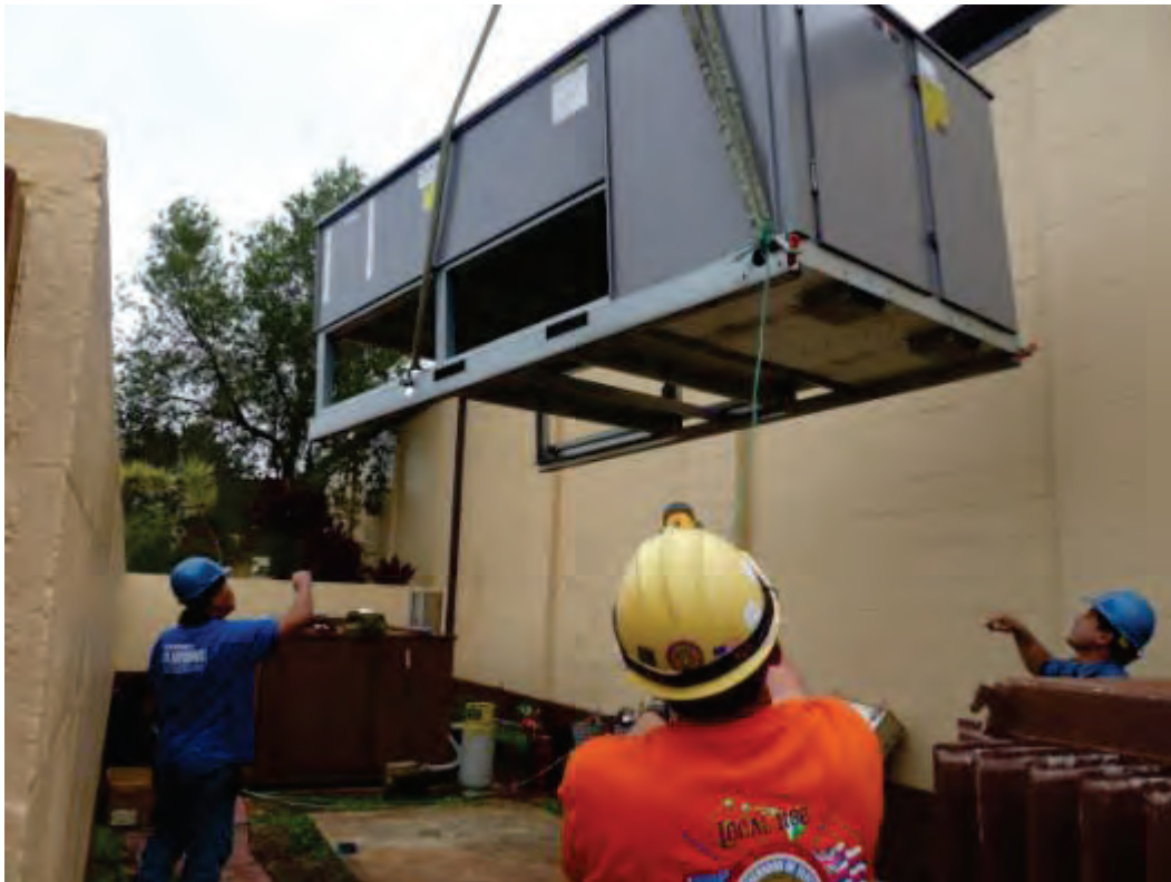
Figure 3. Positioning one of two new condenser units outside Schofield Barracks Bowling Center.
