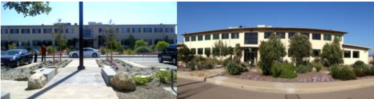
Figure 6. Western façade of Building 6311 before dynamic retrofit (left) and after (right).
