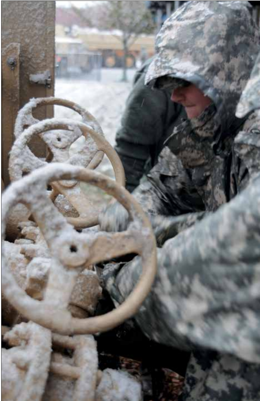
Water purification specialist, part of unit deployed into Rockaway, New York, in direct support of FEMA, state, and local officials, channels water away from housing complex after Hurricane Sandy (U.S. Army/John Adams)
