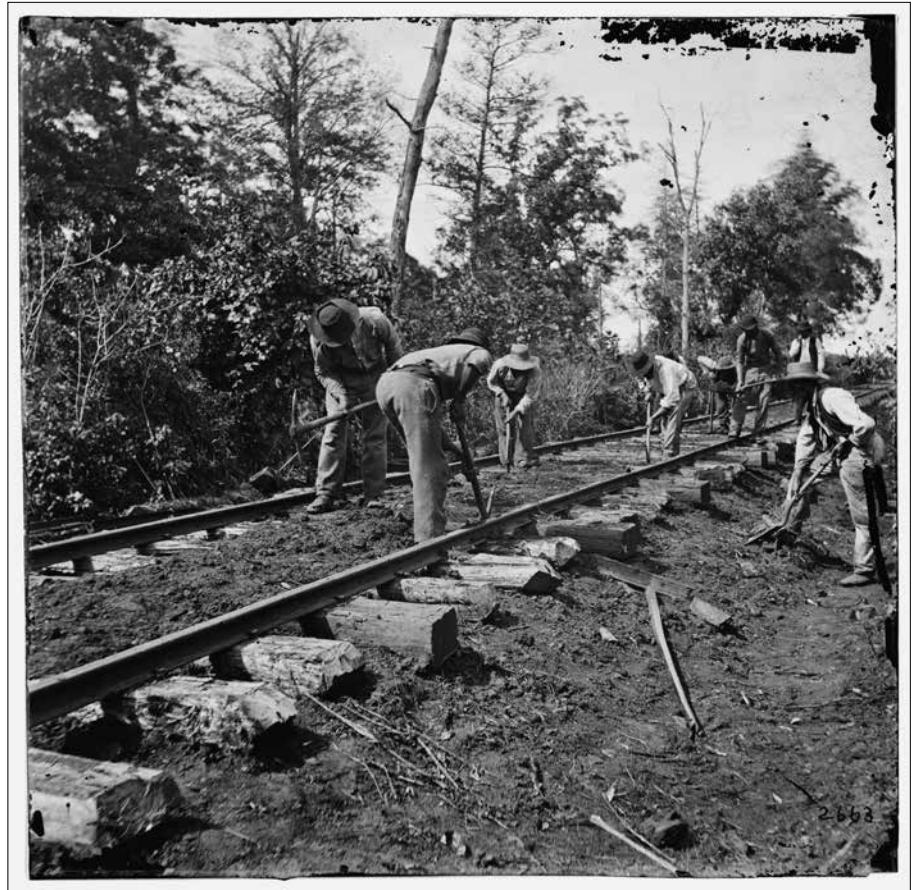
Men repairing single-track railroad near Murfreesboro, Tennessee, after Battle of Stone’s River (LOC)
