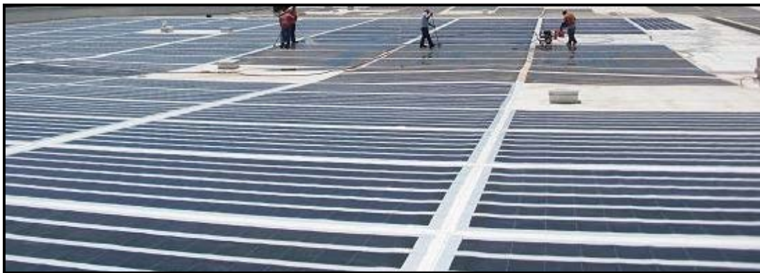
Figure-5: Luke AFB BIPV roof being cleaned during adhesive-failure fix.
