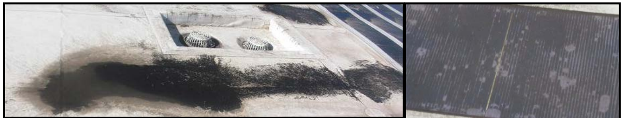
Figure-21: Severe, localized mold growth due to water ponding (left) and PV delamination (right).
