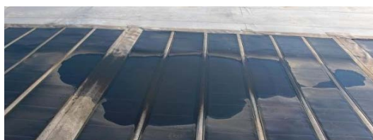
Figure-17: Site II (NAS Patuxent River) water ponding.
