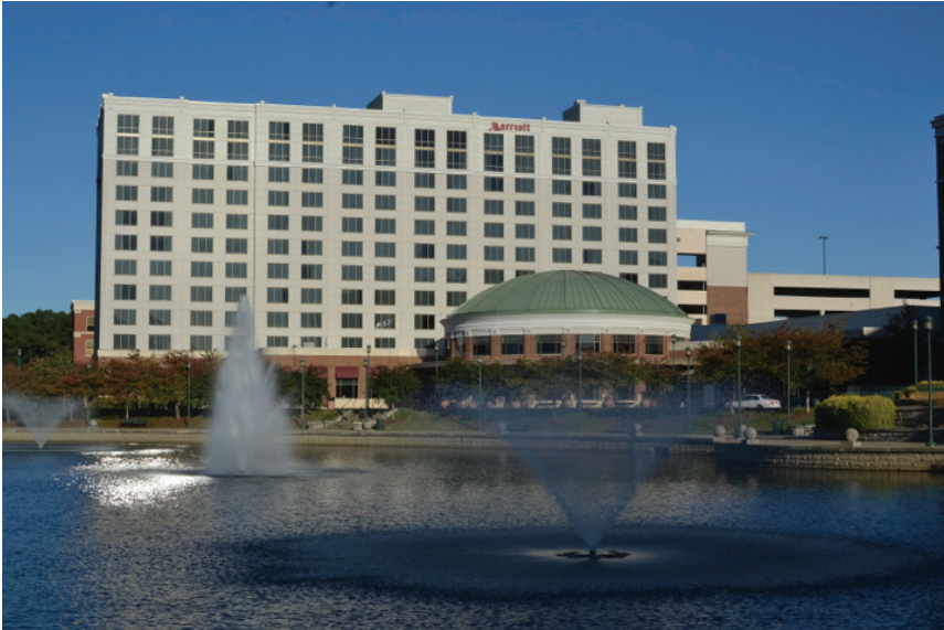
Figure 3.7 Newport News Marriott at City Center
