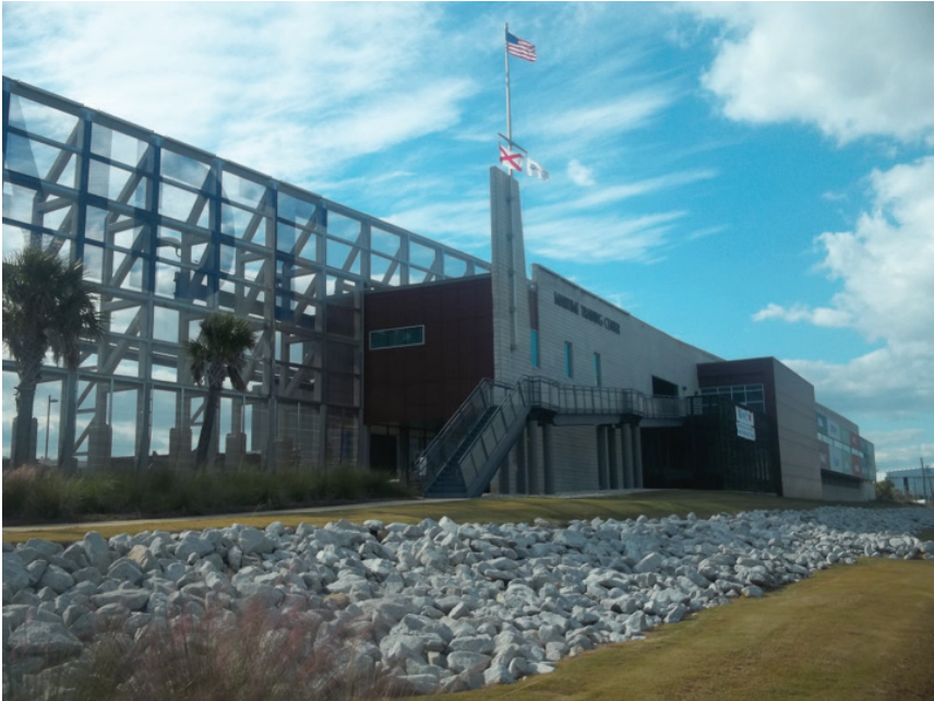
Figure 4.6 Alabama Industrial Development Training Maritime Training Center
