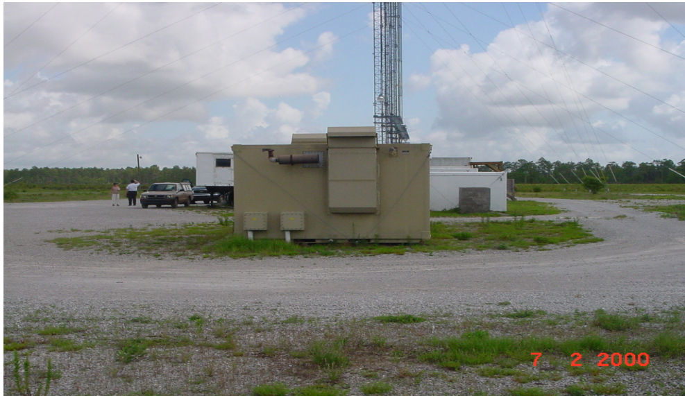
Figure 4 Proposed site for office and equipment facility at A-73 Radar Tower site
