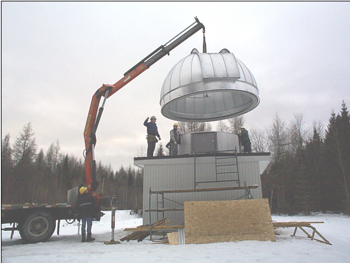
Figure 6. Installation of CASTOR-V's observatory dome in winter 2002
