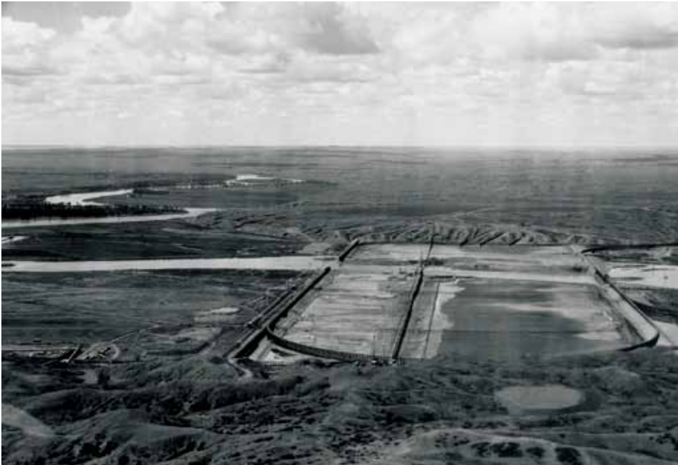
The railroad trestle system outlines the edges of the dam. The cut off wall is under construction down the center of the dam. The section of the river in the left and upper left as well as much of the land are now part of Fort Peck Lake.
