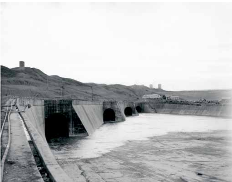
Twenty-nine minutes after the water first entered the tunnel intake portals water flowed out of all four tunnels on the downstream side.
