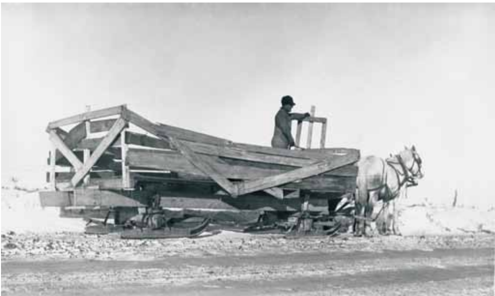
Before the roads and railroad could be built, sleds and horses hauled supplies to the dam site.
