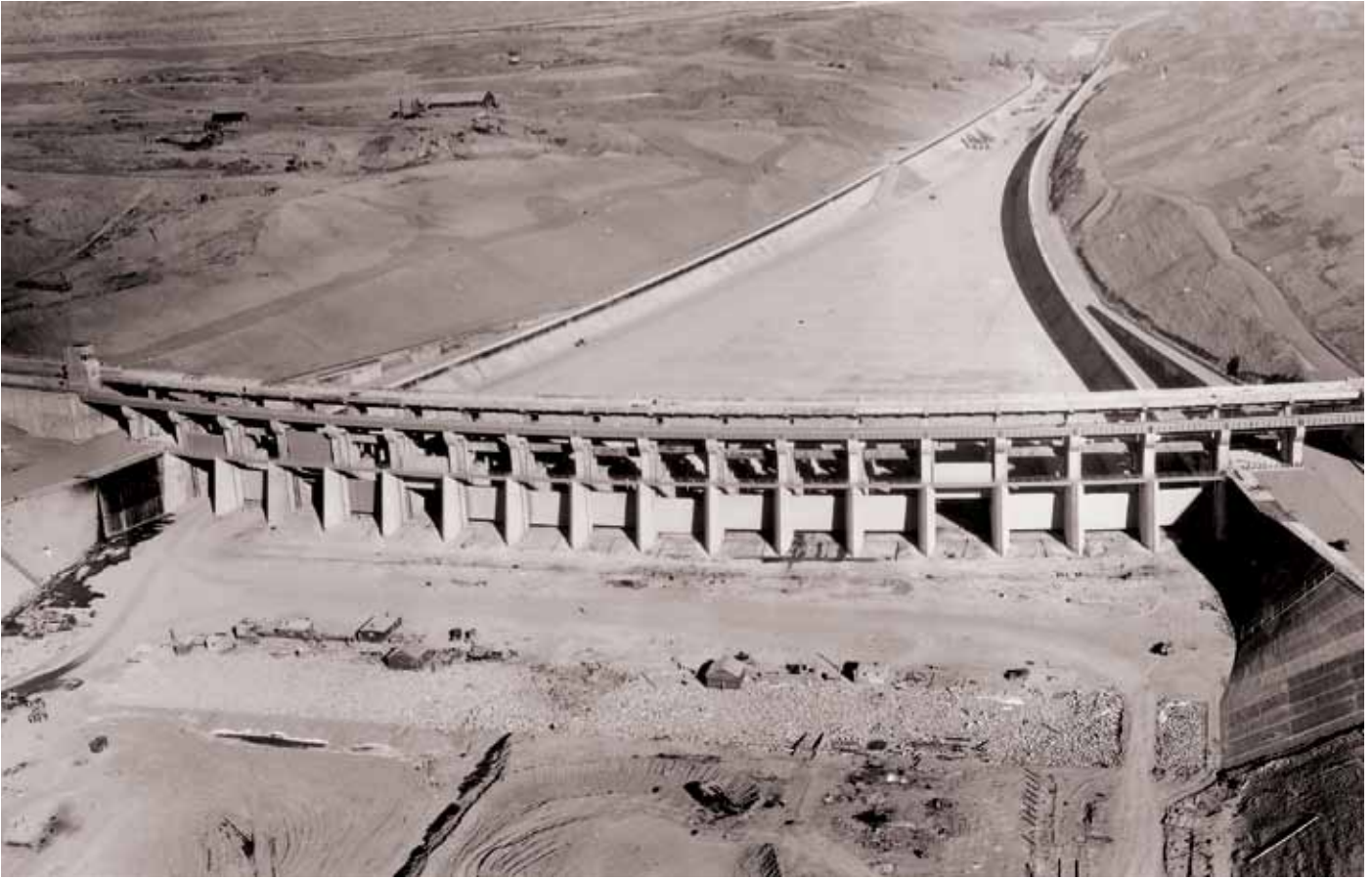
Above: Spillway under construction in 1937.
