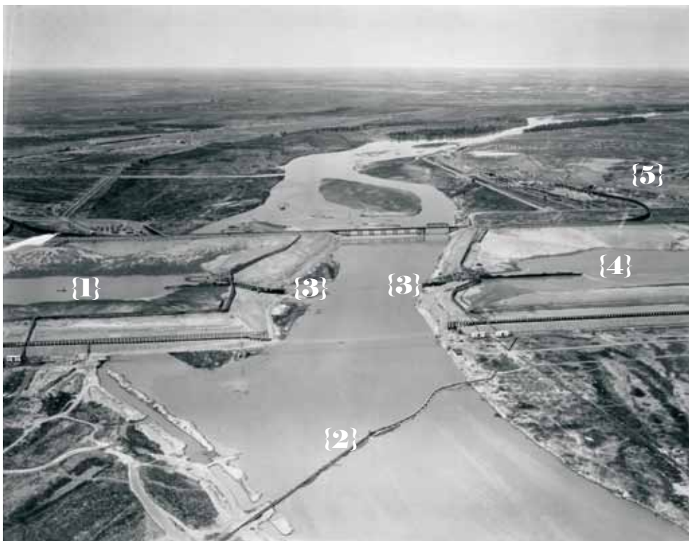
Fort Peck Dam in 1936 showing the west and east core pools with the river open in the center.
