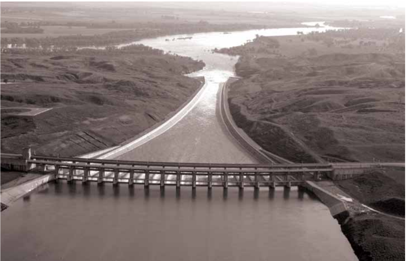
Below: Spillway in use for the 5th time in its history in June 2011 with all 16 gates open. Photo courtesy Valley County Sheriff's Department.
