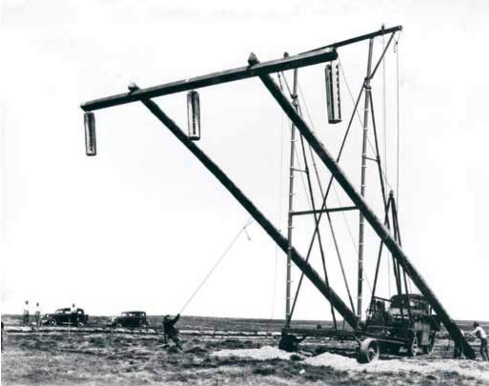
The 288-mile power line took 14 weeks to build and required some 5,500 poles.
