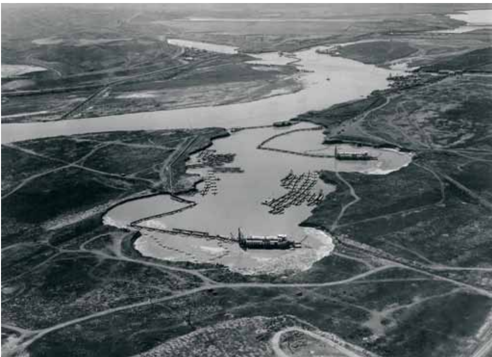
Dredge Jefferson, center, and Dredge Missouri, at right, in foreground. Dredges Gallatin and Madison in upper right background. The dredges pumped the slurry through 28-inch pipelines to the dam in the background. The dredges at Fort Peck set records for both the distance and height that the slurry was pumped.
