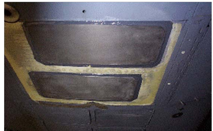
Composite Patch Repair
